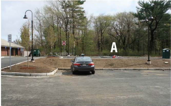
Site Option A fronts an existing parking lot that is expanded to the right. Shared parking between the Senior Center and Town Library is realistic due to the diversity in the time of peak use between the Senior Center and the Town Library.
