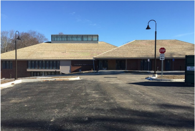
Proximity to Town Library and its parking lot is one benefit of this site as an option for the Senior Center
