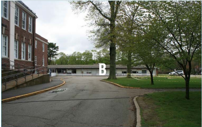
Site Option B locates the new Senior Center where the one story wing is. This site gives the Senior Center frontage onto First Parish Road and creates a New England type of village green with the Gates School, the church, and the water tower across the street.
