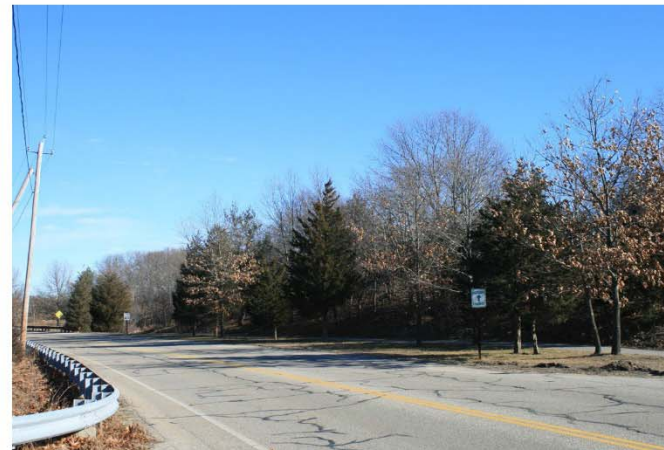
Site along New Kent Street.
