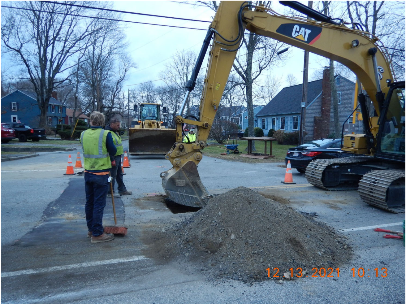
Water Main Replacement
