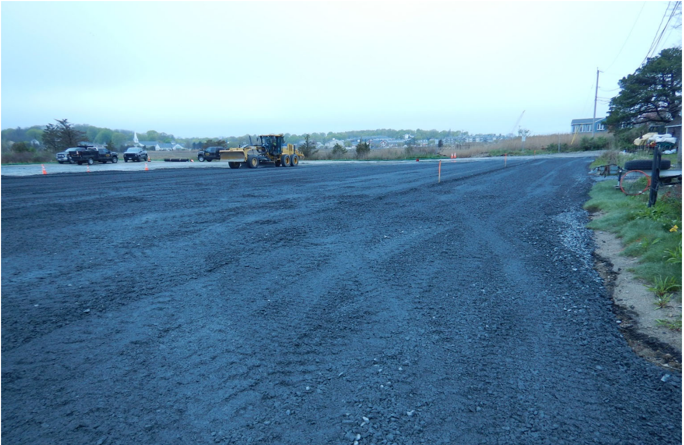
Peggotty Beach Parking Lot Repair Work
