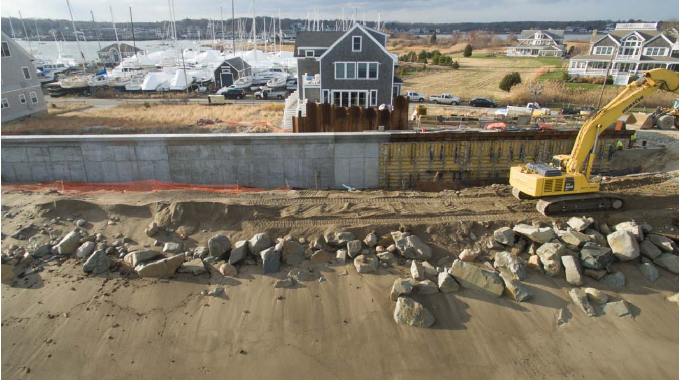
Edward Foster Road Seawall
