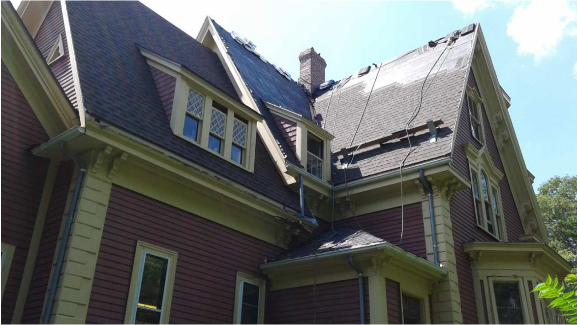
Bailey Ellis House Roof
