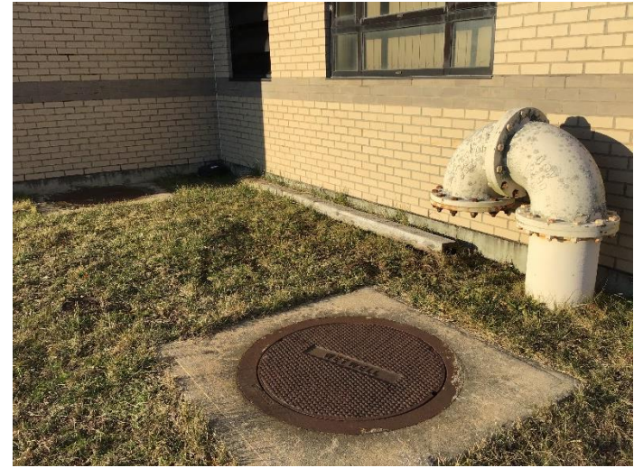
Photo 12 Instrumentation Manhole in Front of Filter building
