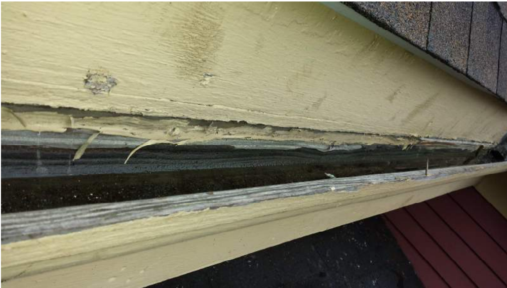
Sealant on original wood gutters in need of replacement Phase III
