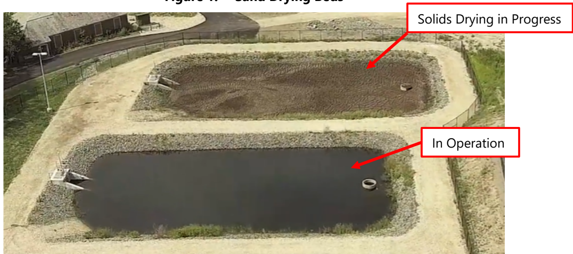
Figure 1: Sand Drying Beds
