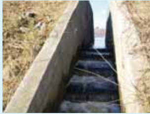
Fishway exit channel modifications
