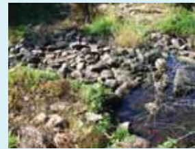
Fishway entrance channel improvements
