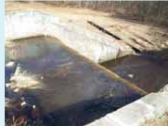
Spillway bottom hinged crest gate
