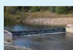
Modifying dam outlet
