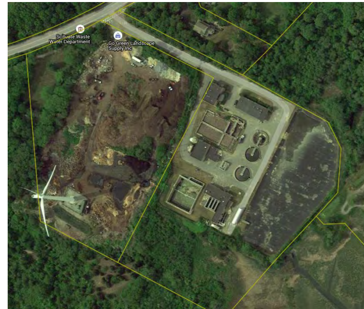
Scituate Wastewater Treatment Plan on the Driftway
