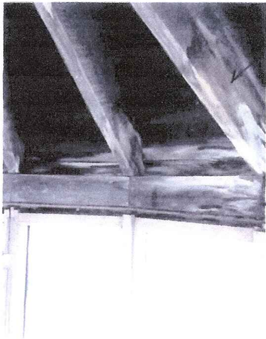
Interior view Lighthouse lantern windows and roof framing
