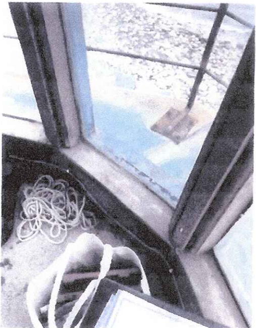
Interior view Lighthouse lantern windows and concrete floor slab
