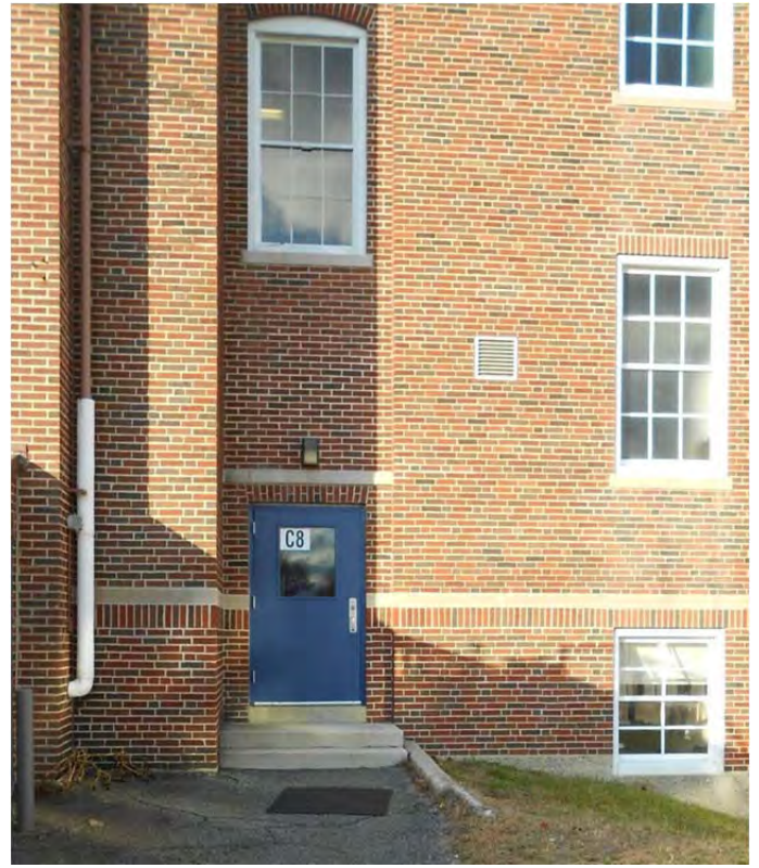
South elevation, eastern door at exit stair.
