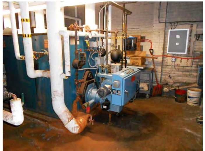
Painted concrete floor in the basement boiler room.
