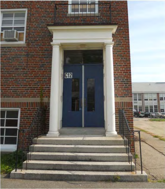
Portico elements of west elevation fabricated of GFRP.
