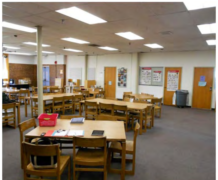
View of suspended ceiling in library area with standard acoustic tiles.
