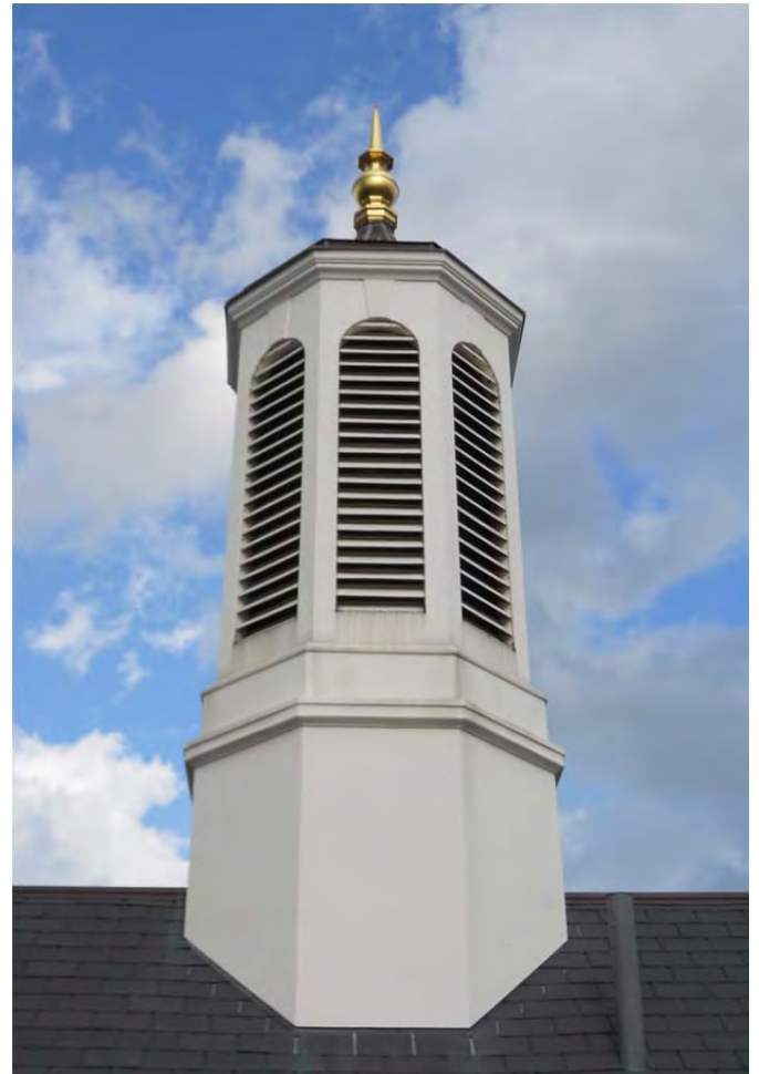
Cupola fabricate of GFRP with restored gilded finial.
