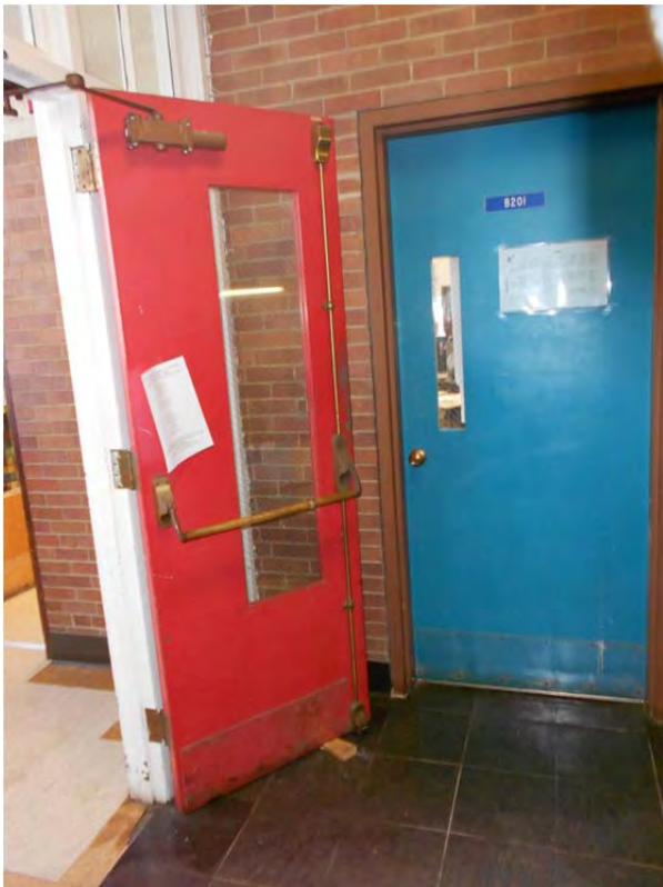
Typical metal door at exit stair.
