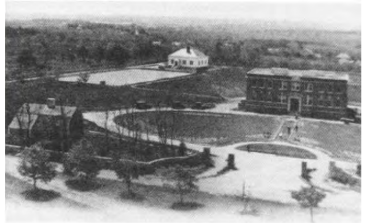
Original building constructed in 1917 with flat roof.
