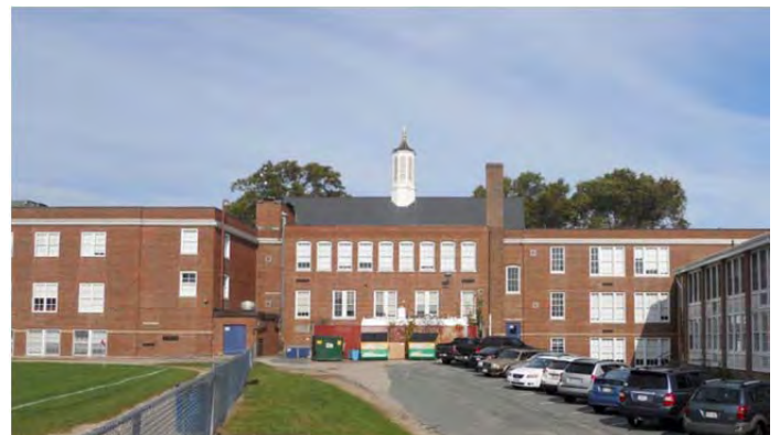
South elevation of existing school.
