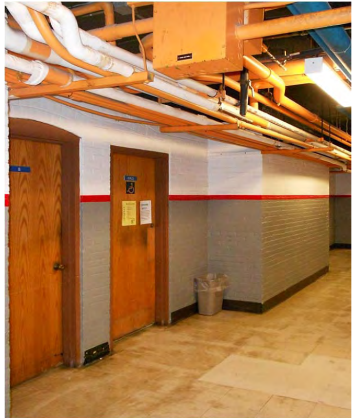
Typical basement corridor of original building with painted brick.
