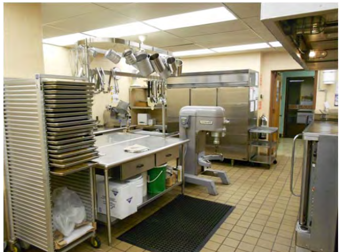
Ceramic tile floor in the basement kitchen area.
