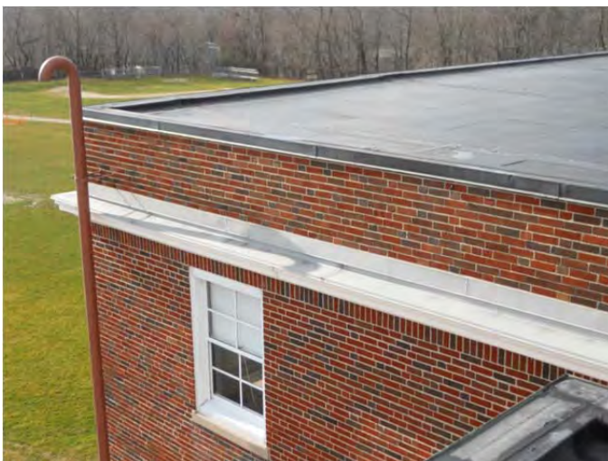
Band course fabricate of GFRP at west wing.
