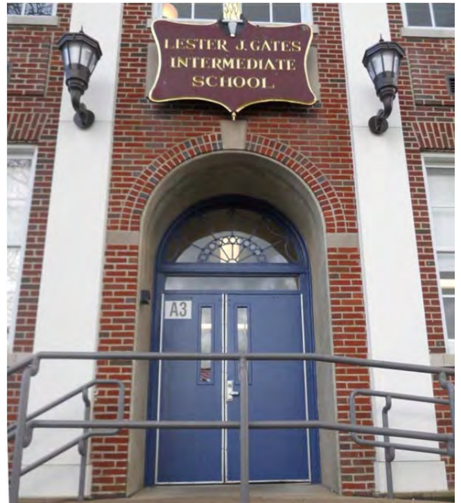
Main building entrance with original fanlight remaining.
