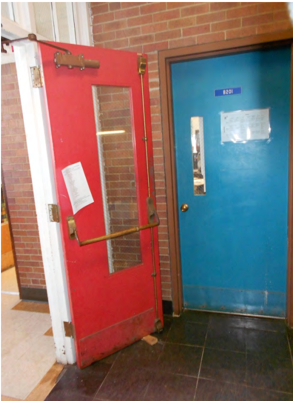
Typical metal door at exit stair.
