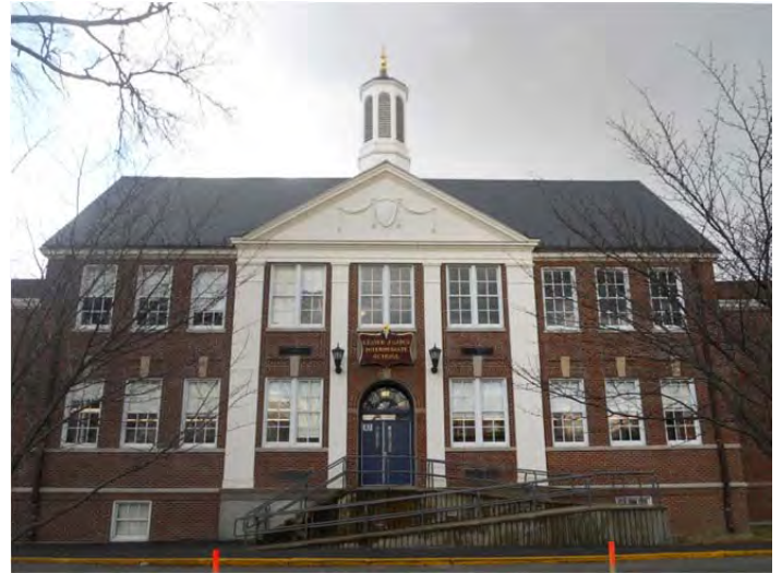
Current state of building with synthetic roof slate, January 2012
