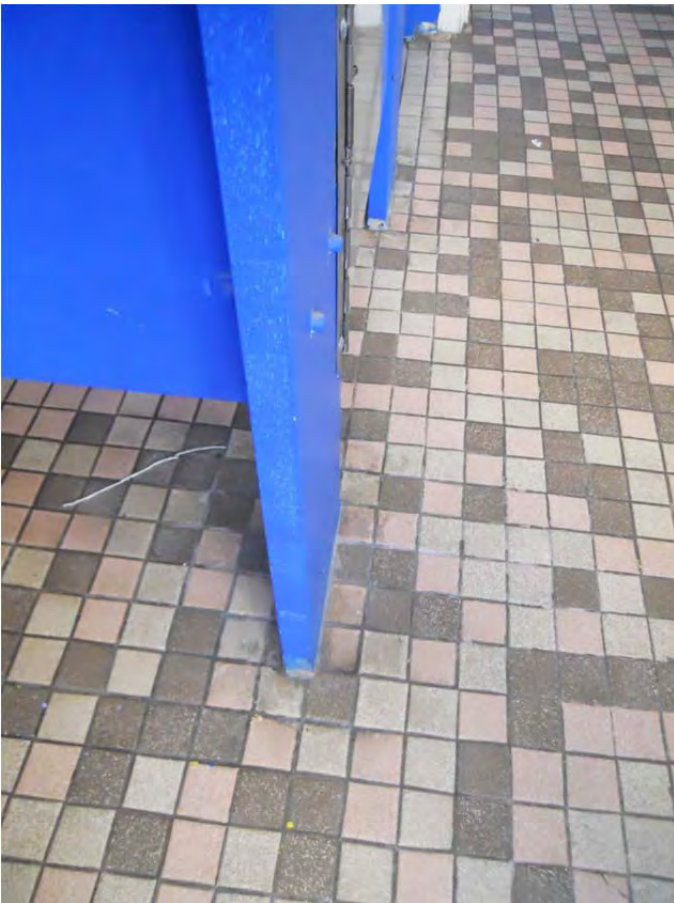
Typical ceramic tile floor in restroom areas.
