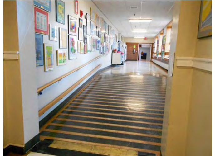
Ramp transition between original building and west wing at first floor.
