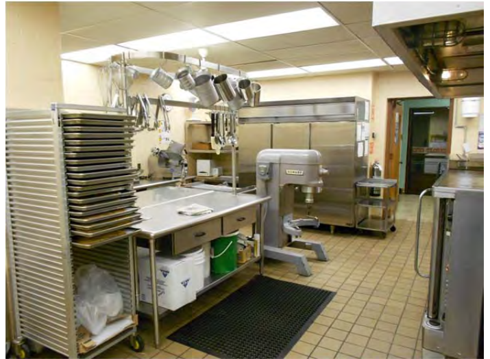
Kitchen ceiling with metal panels.
