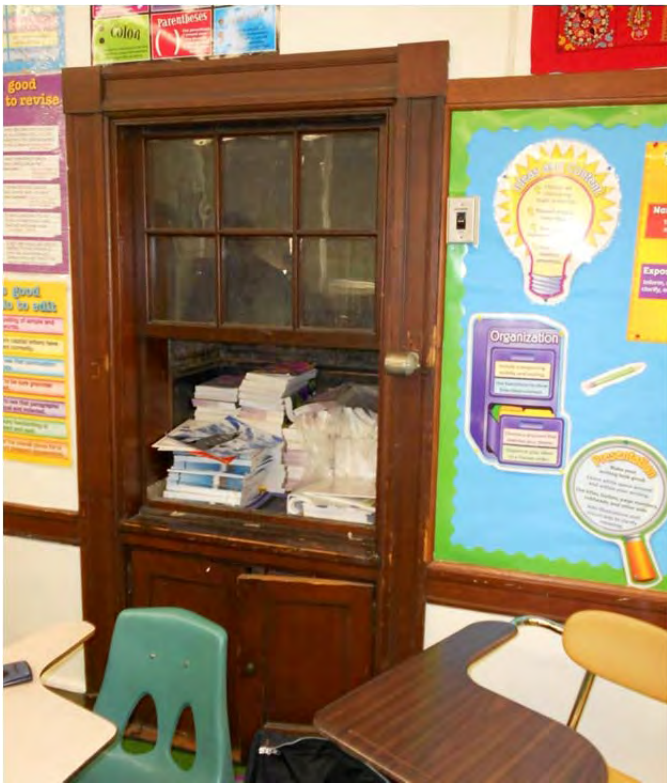
Original built-in casework with fume hood remaining in original building.
