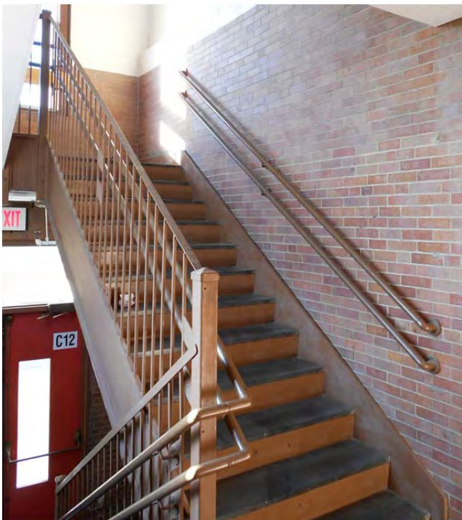
Exit stair at southwest corner of the west wing.
