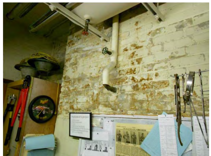
Painted masonry walls in basement utility areas.
