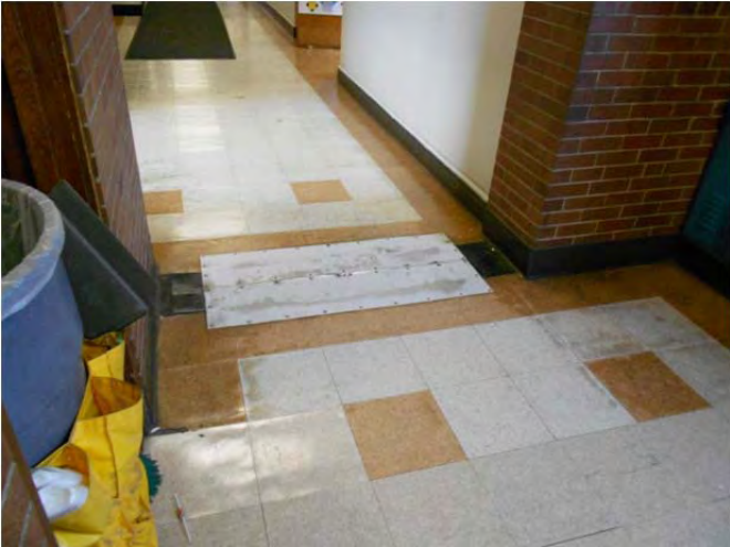
Corridor floor transition between original building and XXXX wing.
