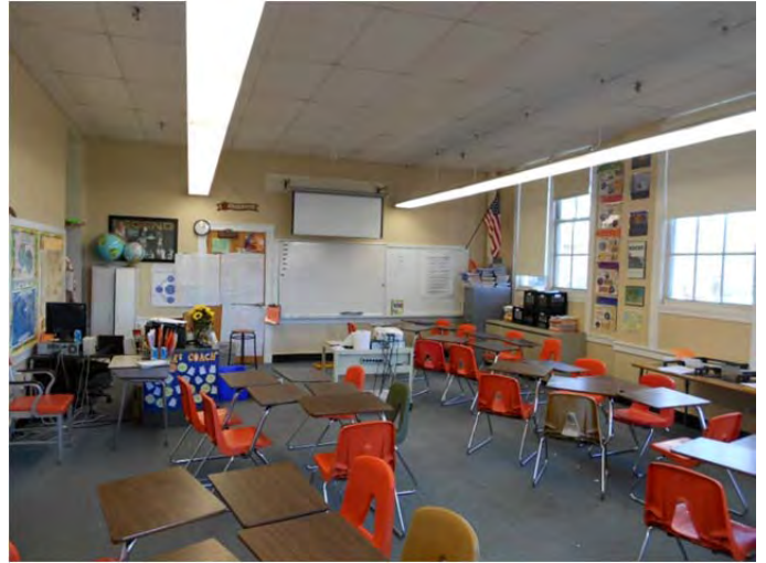
Carpet at a first floor classroom.
