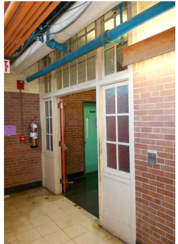
Historic frame with transom and sidelights at stair.
