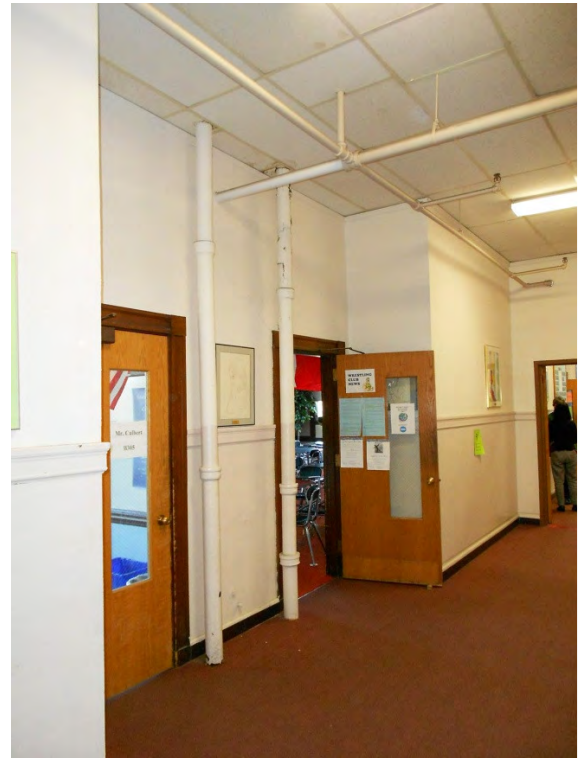
Typical wood classroom door.
