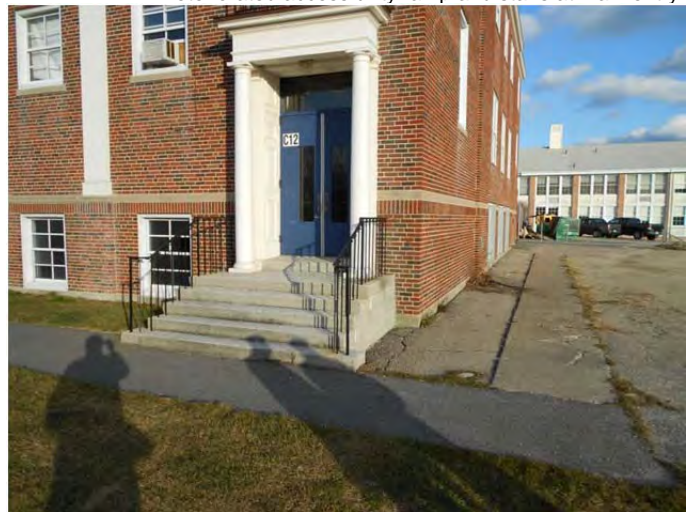
Exit door and stairs at west elevation of west wing.
