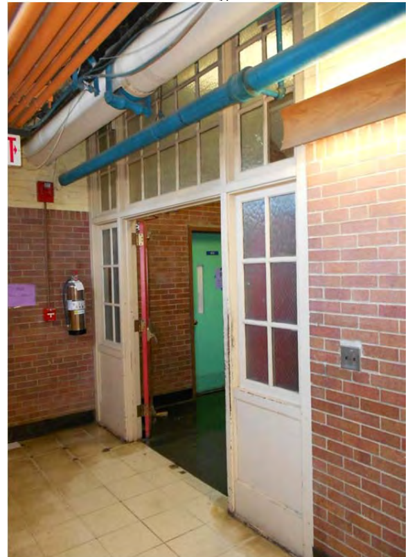
Typical historic frame with transom and sidelights at exit stair.
