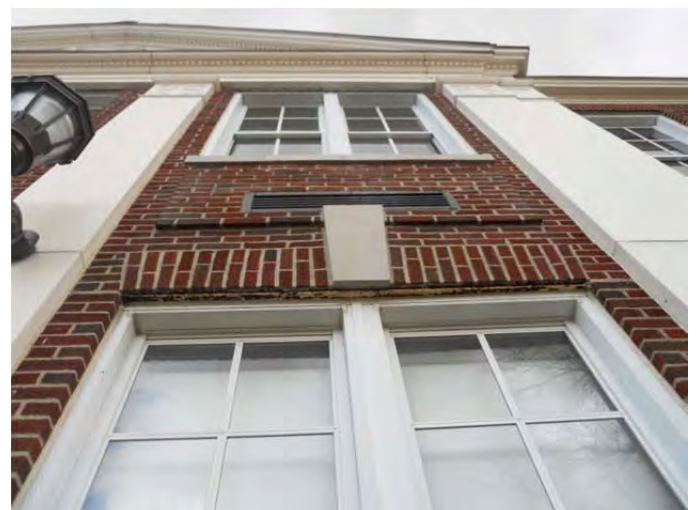
Main entry elements fabricate of GFRP such as pilasters and pediment.
