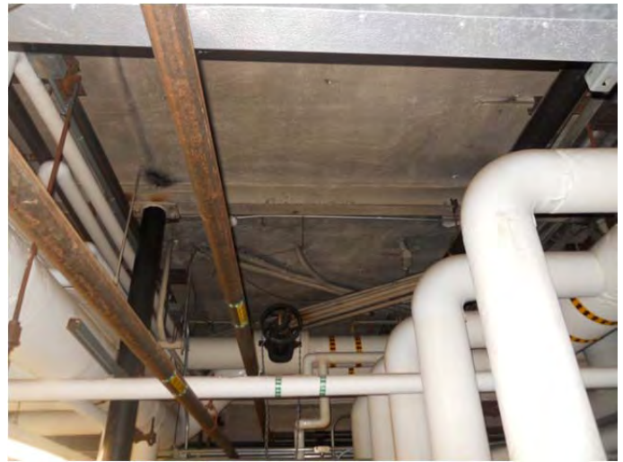
Original plaster ceiling remaining in boiler room of basement.
