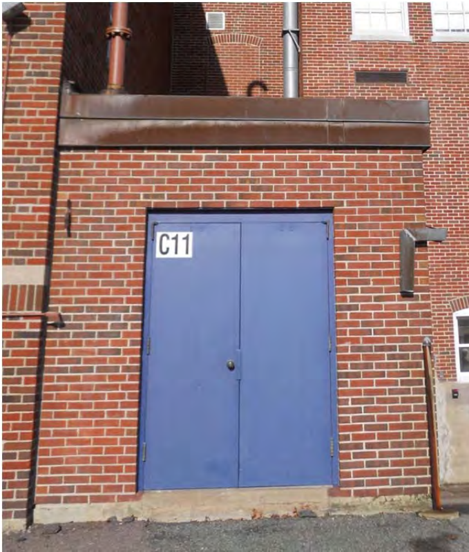
South elevation, western door at utility enclosure.
