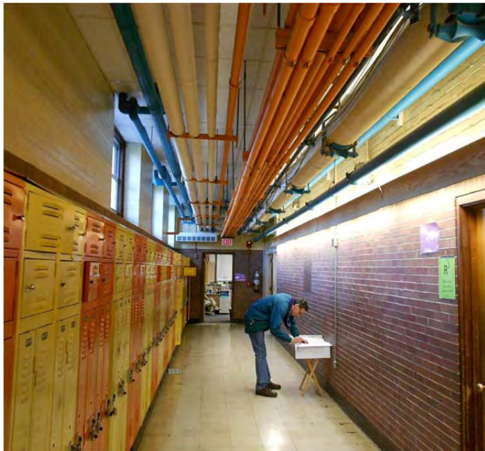
The amount of lockers and adjacent classrooms create congestion.
