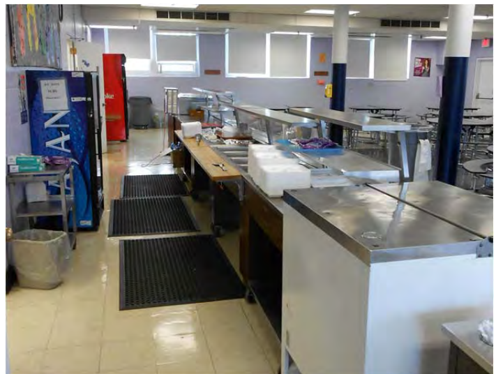
The serving equipment is located outside in the kitchen in the cafeteria.
