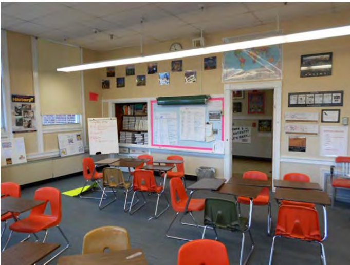
Painted plaster walls in the original building.
