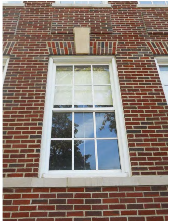
Typical metal replacement window.
