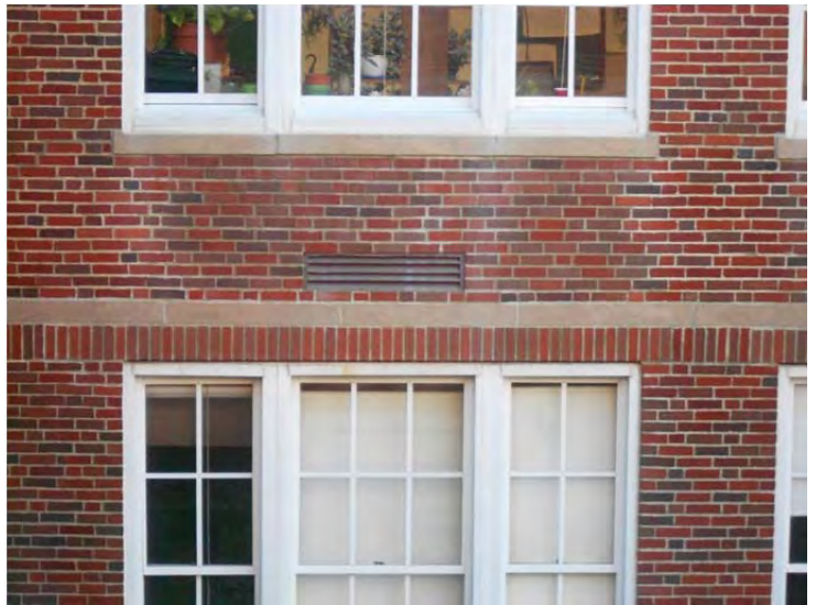
Louver at east elevation of east wing.
