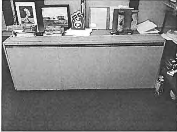
Floor-mounted unit ventilator
