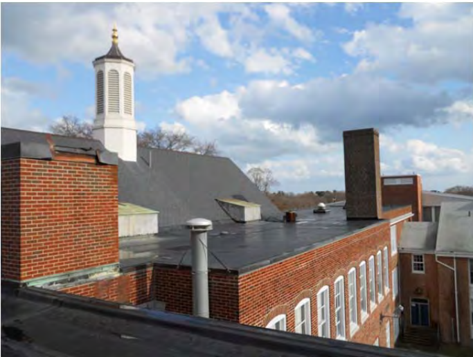
Flat roof at east, south and west sides of original building
