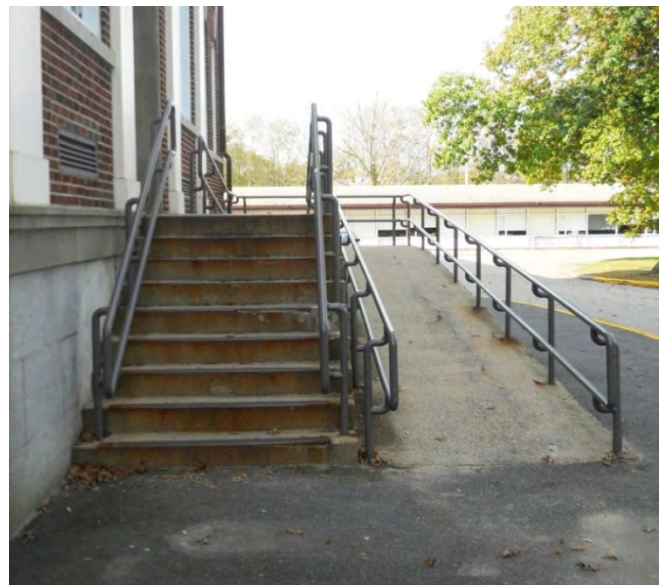
Main entry ramp and stairs.
