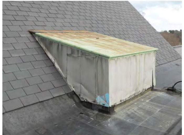
Shed at south side of original building housing HVAC equipment.
