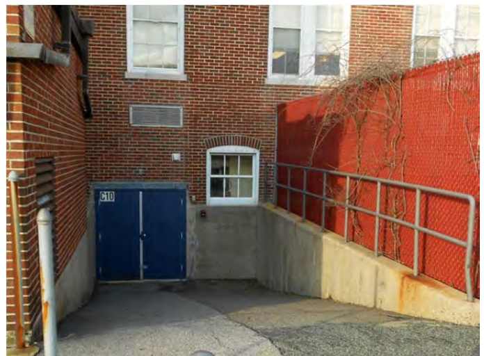
South elevation, central service doors to basement.
