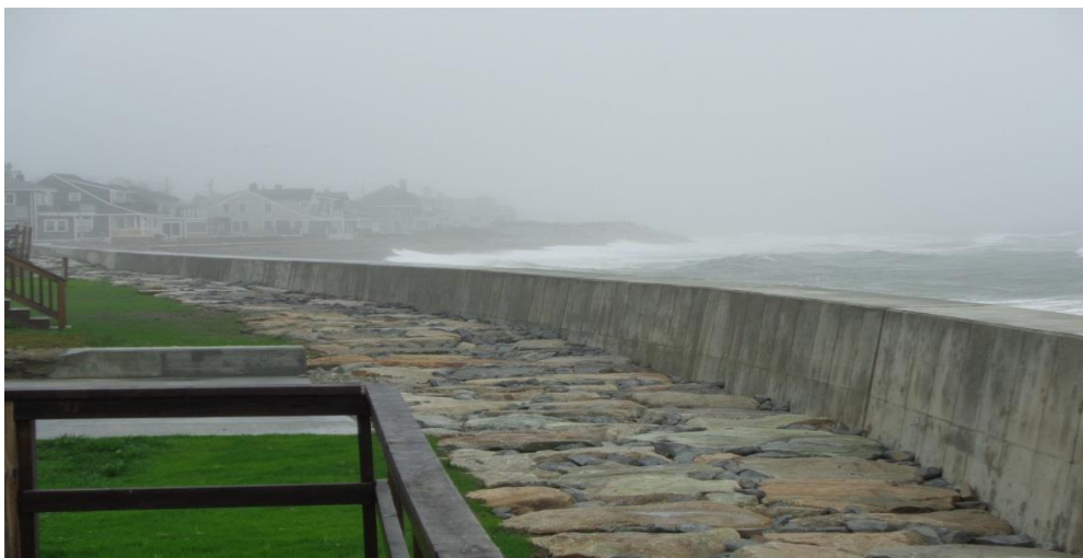
Splash Pad at Oceanside Drive Seawall, photo credit Kevin Cafferty
