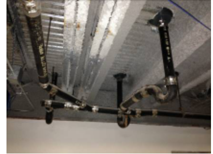
Addition Drainage Piping
