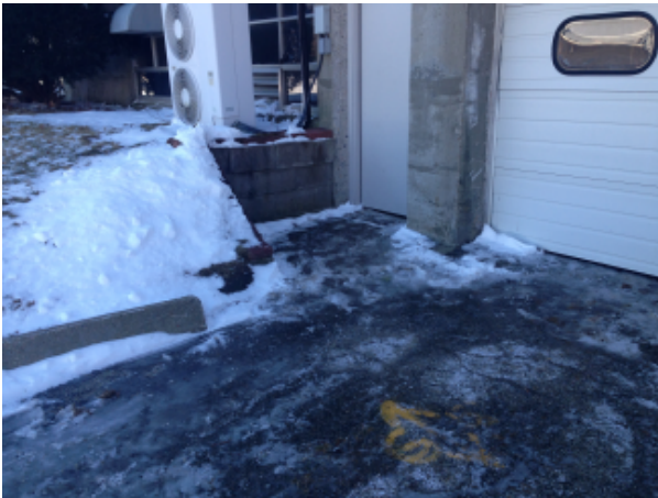
Figures 1 & 2: Paint within driveway north of Town Hall and walkway south of Police Station indicating gas services
