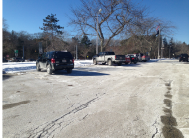
Figures 4 & 5: Cracked and degraded pavement in north parking lot and cracked pavement in south parking lot.
