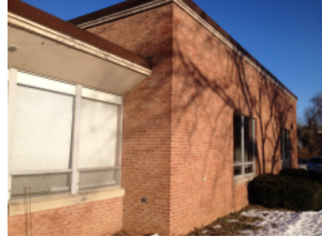
Exterior Brick Veneer and Windows
