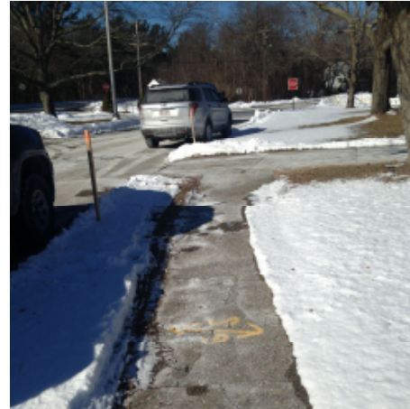
Figures 1 & 2: Paint within driveway north of Town Hall and walkway south of Police Station indicating gas services
