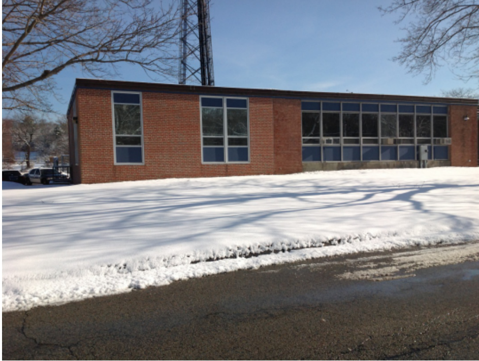
Scituate Police Station
