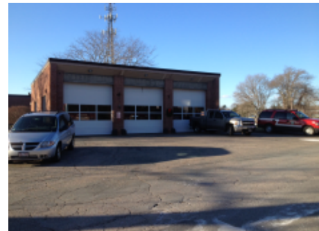
Apparatus Bays - Overhead Doors
