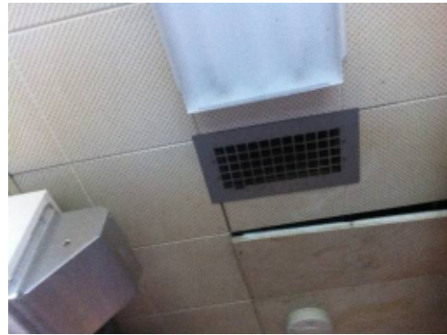
Cell Transfers and Ceiling General Exhaust
