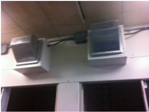
Cell Transfers and Ceiling General Exhaust
