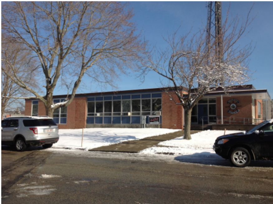
Scituate Police Station
