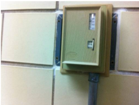
Pneumatic and Programmable Thermostats
