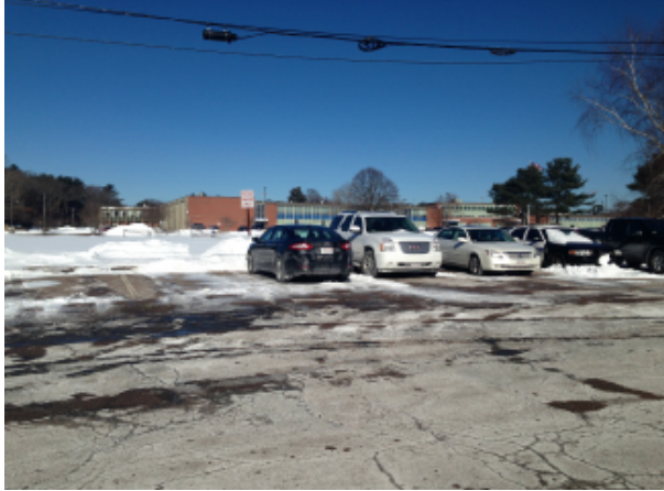
Figures 4 & 5: Cracked and degraded pavement in north parking lot and cracked pavement in south parking lot.
