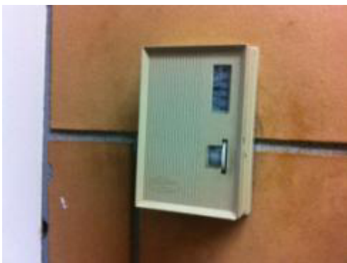
Pneumatic Thermostat and Pneumatic Control Valve
