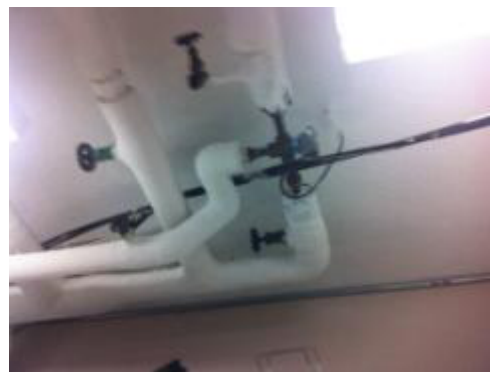
Pneumatic Thermostat and Pneumatic Control Valve
