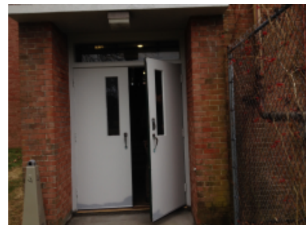
Typical Exterior Doors
