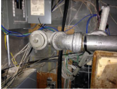
Original Bldg Drainage Piping
