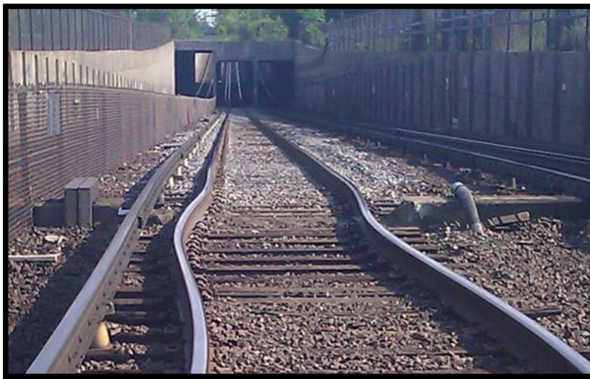
Figure 28 Heat kink on MBTA track.
