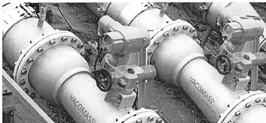
Figure 9 – Binder Vacomass Jet Valve (Courtesy of Binder)
