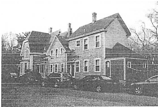
3. Southwest and southeast facades (L to R: Main House, Middle Addition, End Building Addition, Shed)
