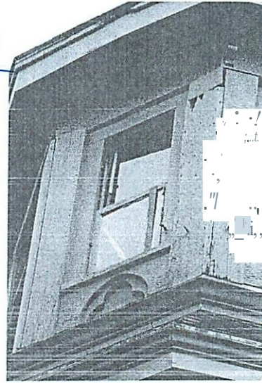
47. Northeast fac;;ade - Tower detail: broken glass; deteriorated wood trim
