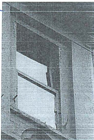
49. Northeast façade - Tower detail: Deteriorated wood trim
