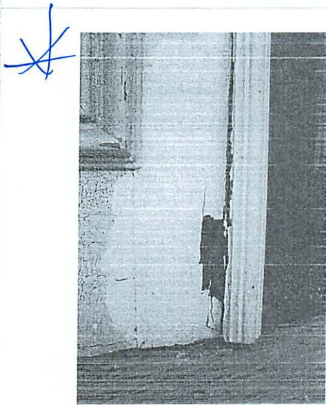
21. Main (southwest) façade - Main entrance door: deteriorated stile
