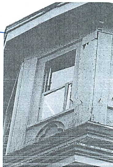
48. Northeast façade - Tower detail: broken glass; deteriorated wood trim
