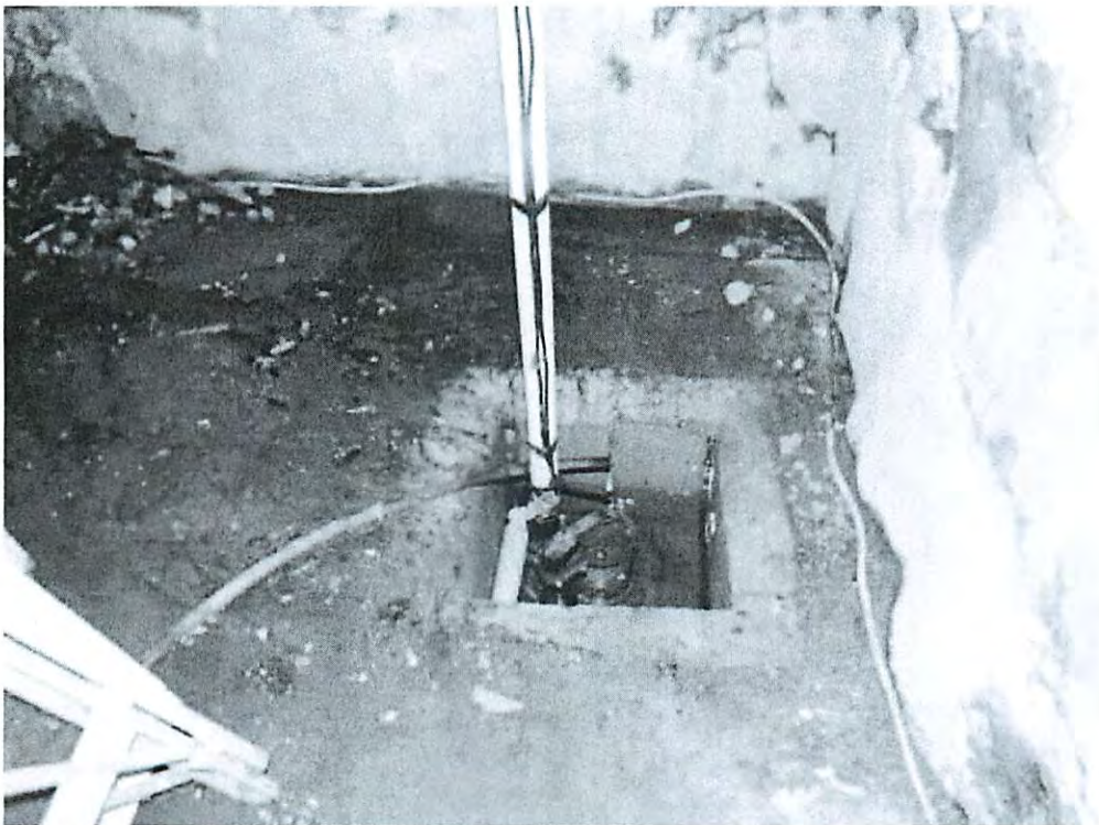
Photo of existing sump in basement-A
