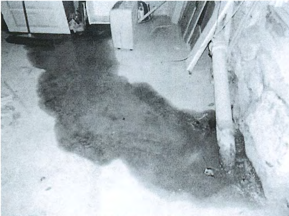
Photo of north foundation wall in basement - B
