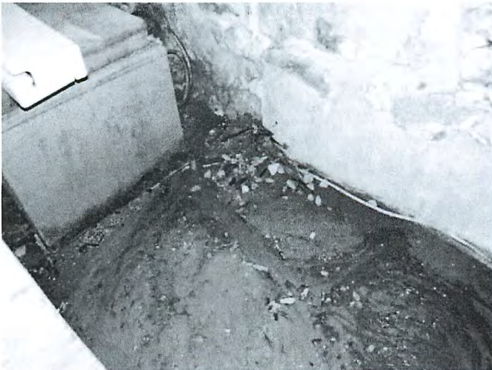
Photo of south foundation wall in basement - C
