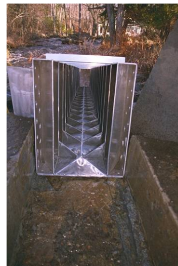
Fig. 6. Alaskan steeppass fish ladder at Unicorn Lake, MD (left). Upstream exit of Alaskan steeppass fish ladder, looking downstream, in the Parker River, MA (right).
