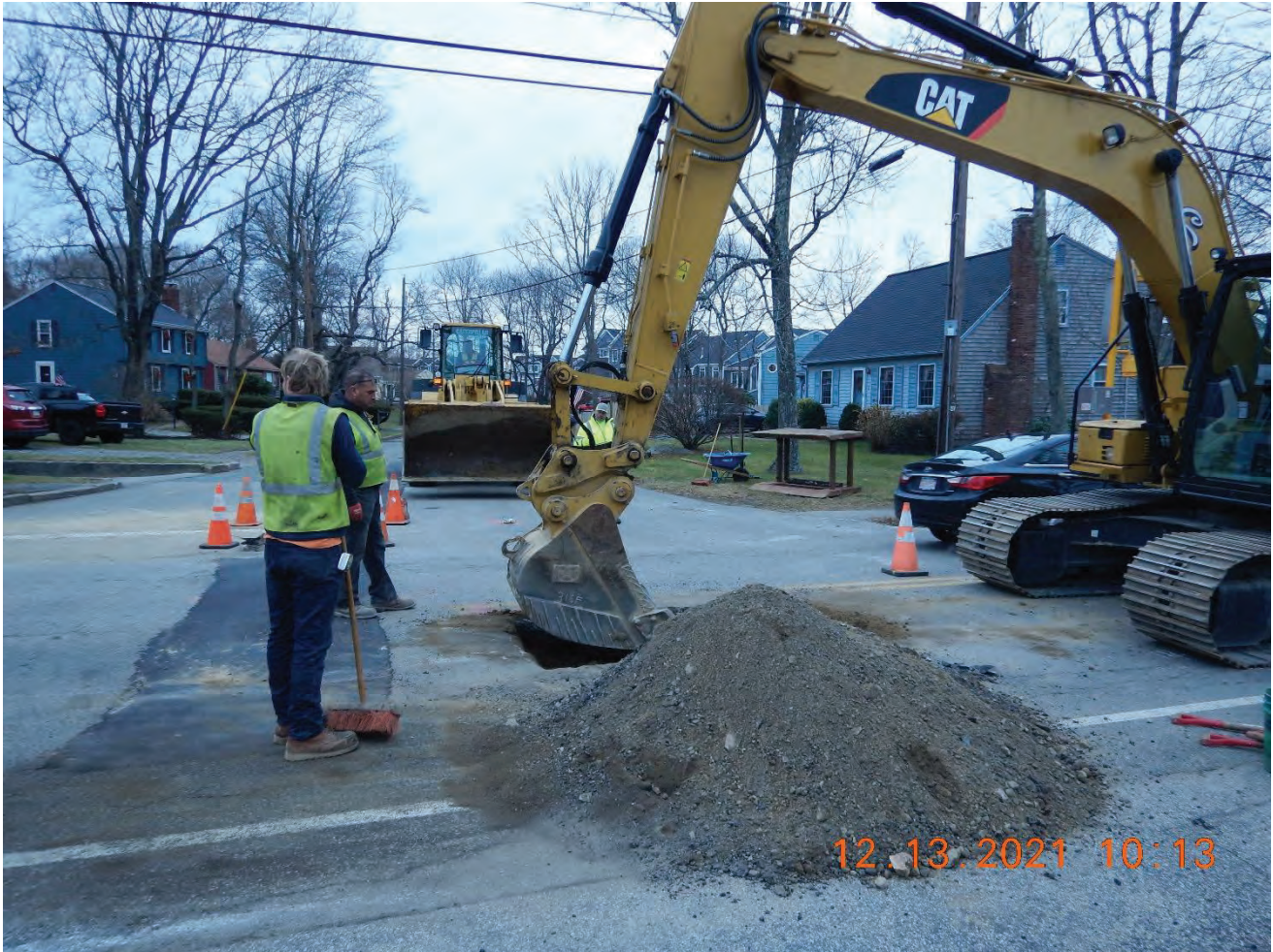
Water Main Replacement
