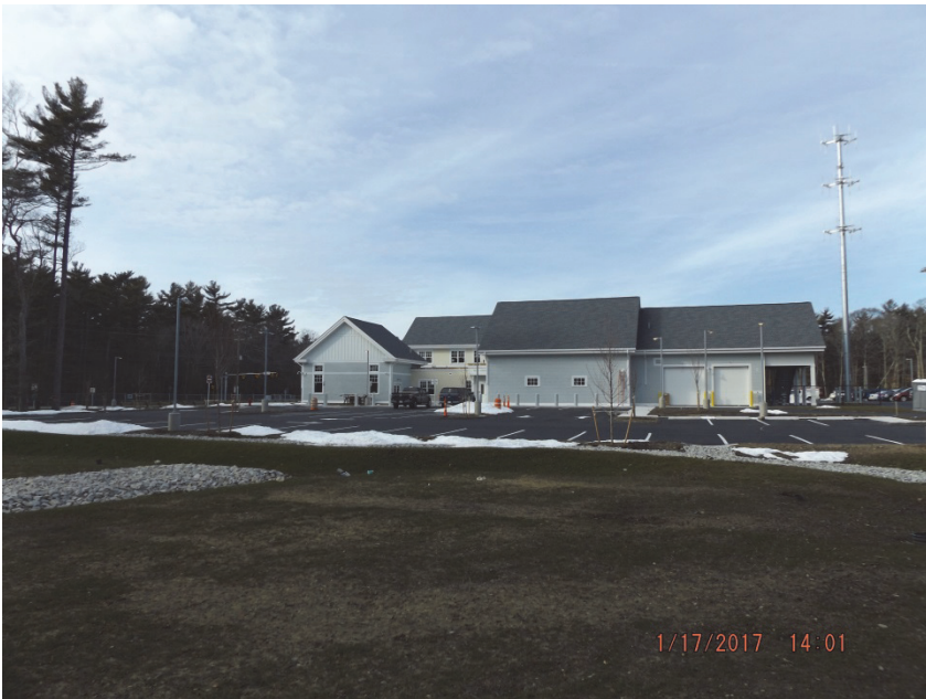
Public Safety Complex as of 1/17/17 (south side facing Mann Lot Rd.)
