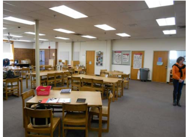
Columns added in Resource Center to support new second floor infill (1974 renovation).
