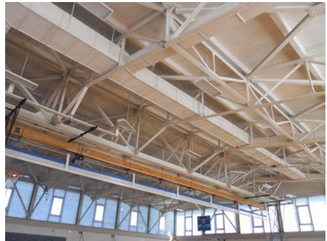
Structural wood decking, wood purlins, and clear span steel roof structure at gymnasium roof.
