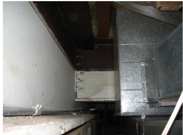
Clear span steel girders over original gymnasium (currently the Learning Center).
