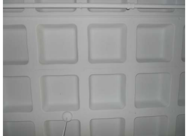
Two-way, reinforced concrete waffle slab system at second floor (gymnasium).
