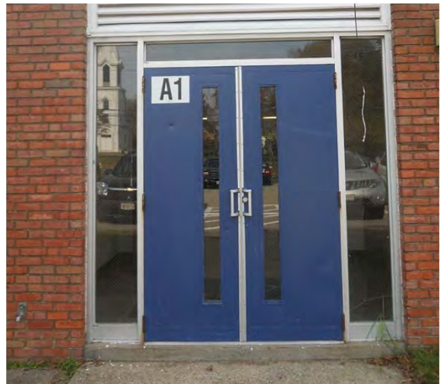
Even on-grade C-wing isn't handicapped compliant with a step down at the egress door.
