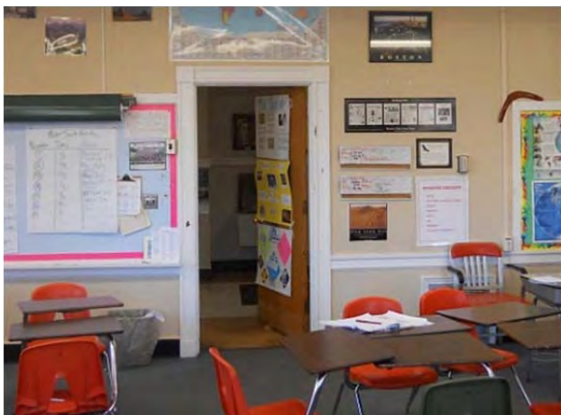
Original casing in B wing
