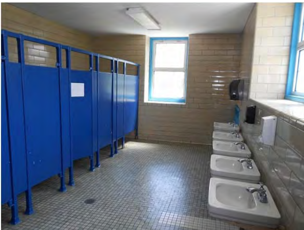
A restroom in A wing that has not been modified to meet handicapped codes.
