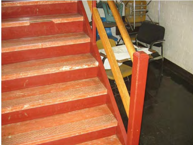
Non-compliant guardrails
