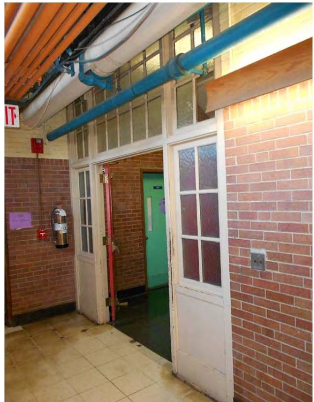
Original unrated stairway frame and glass in B wing
