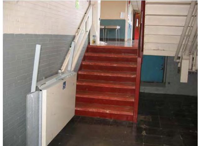
The handicapped lift impedes the stair width
