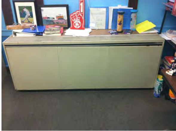
Floor-mounted unit ventilator
