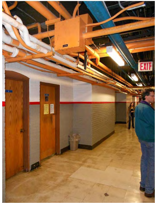
CMU walls in the basement of B wing
