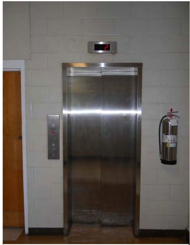
Elevator added to B wing in the 1970s
