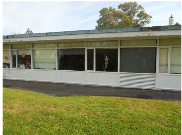
Original wood window system at C wing
