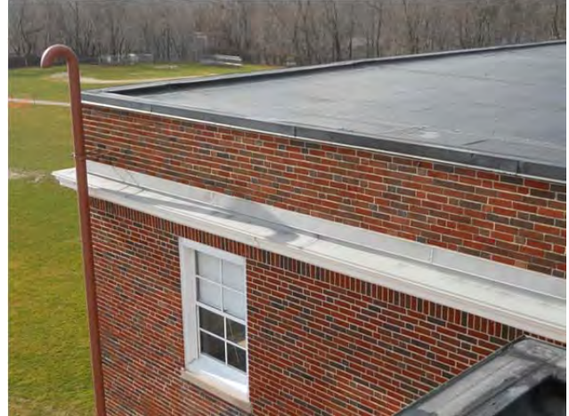
Band course fabricated of GFRP at B wing
