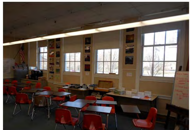
Typical room interior with large windows providing natural light
