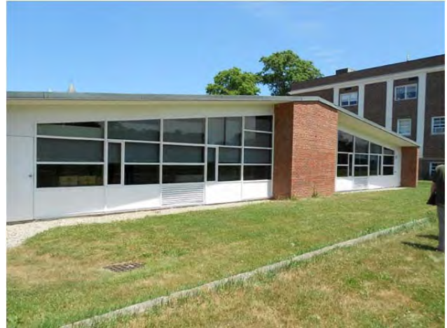
Original wood window system at C wing with non-tempered plate glass facing ball fields
