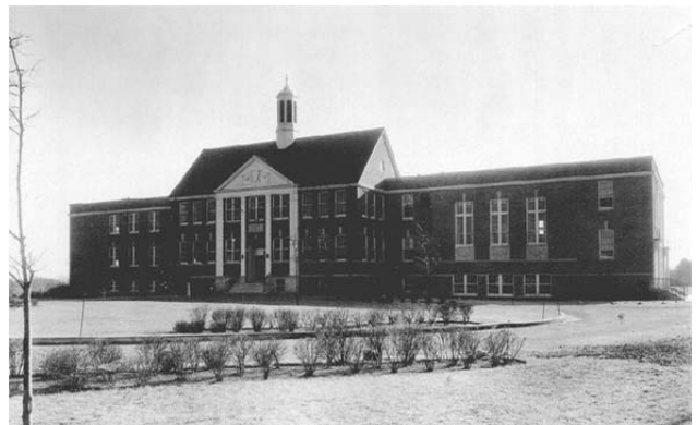
The pitched roof, portico ornament, east wing, and west wings were constructed in 1930.
