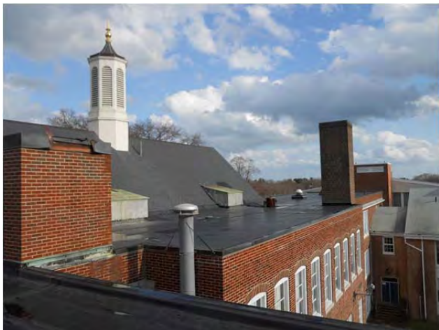
Flat roof at east, south, and west of B wing.
