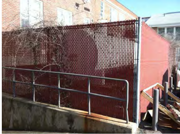
Oil tank behind the enclosure
