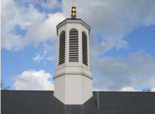
Cupola fabricated of GFRP with restored gilded finial
