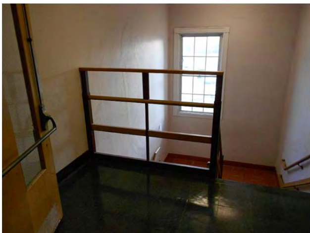
Some existing guardrails have few or no balusters
