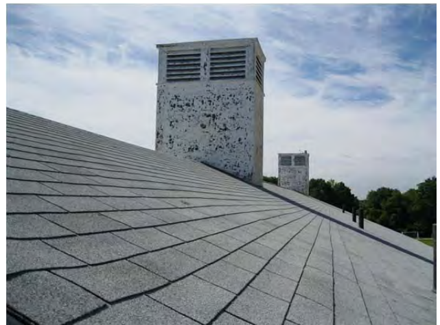
Classroom wing ventilation cupolas
