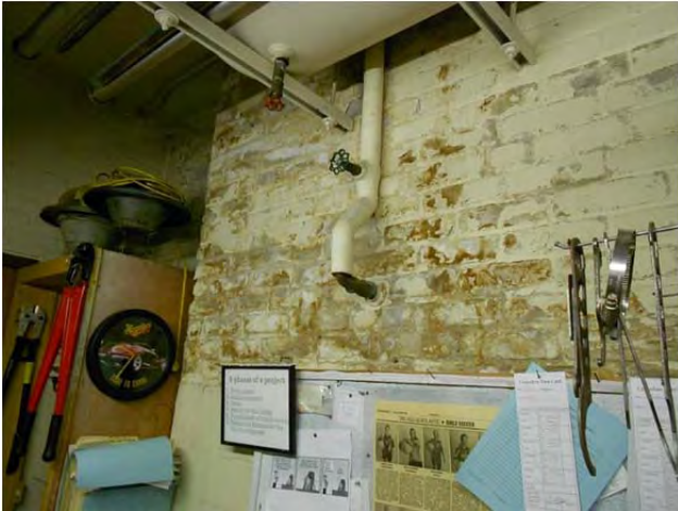
Painted masonry walls in B wing's utility areas.
