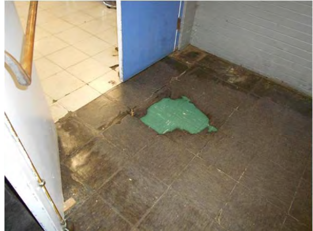
Vinyl tile floors are heavily worn and far beyond their useful lives
