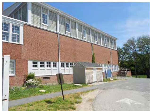
A wing brick walls showing recent repointing
