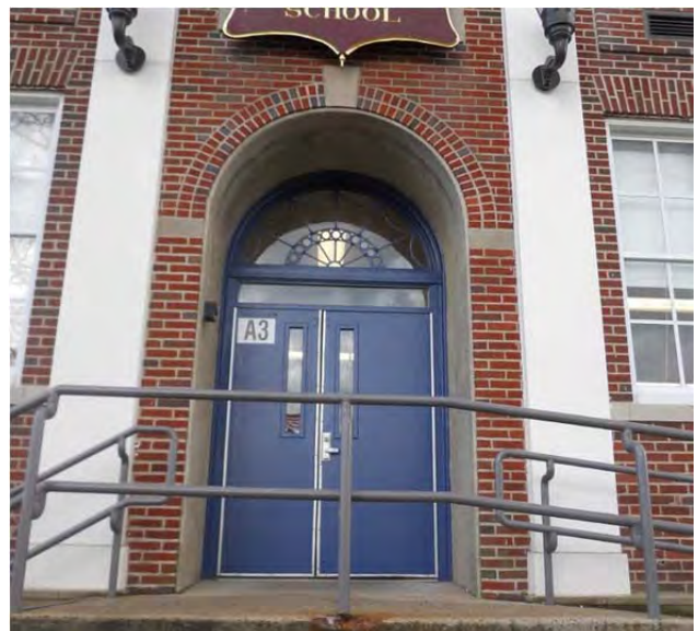
Main entrance located in B wing with original fanlight remaining
