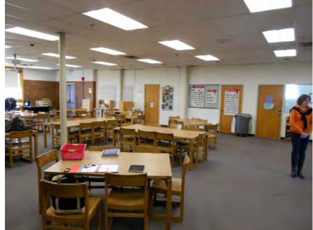
Columns added in Resource Center to support new second floor infill (1974 renovation).
