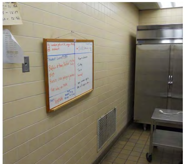
Ceramic tile wall finish in kitchen.
