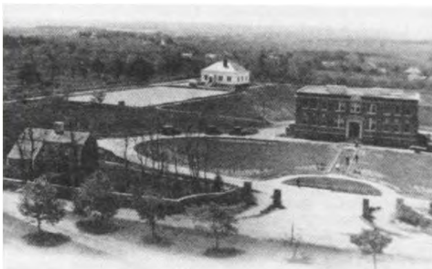
The original building constructed in 1917 with a flat roof. Currently this is the center of B wing.
