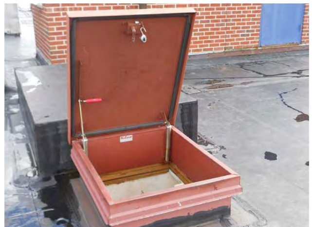
Roof hatch in B wing
