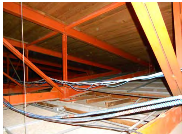
Structural wood decking on typical cantilevered roof trusses at C-Wing.
