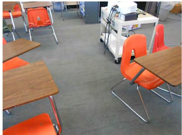
Classroom carpets are stretched, causing ripples, tears, pulls, and tripping hazards.
