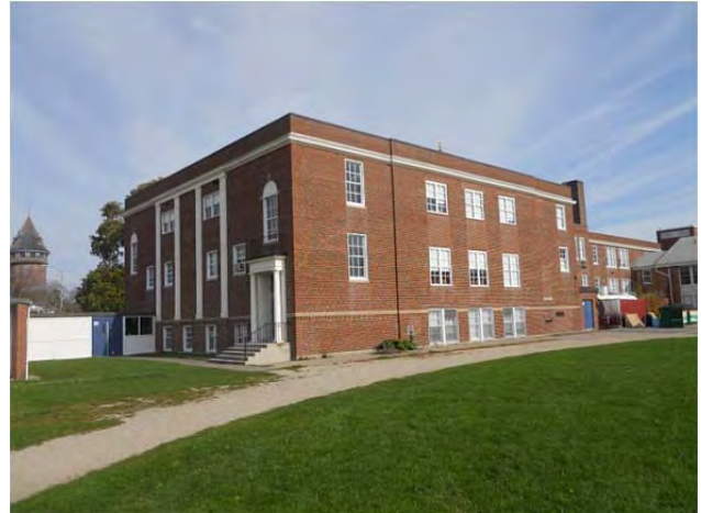
South and west elevations of B wing
