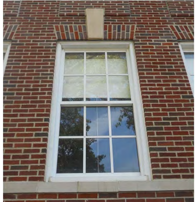
Typical metal replacement window for A and B wings
