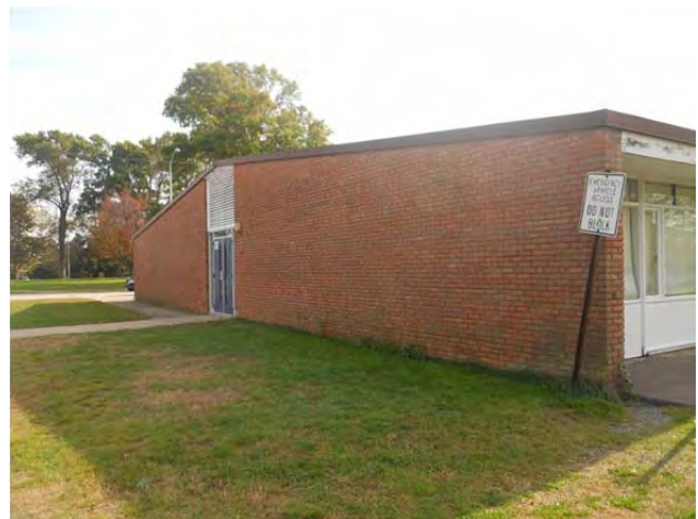
North elevation of C wing
