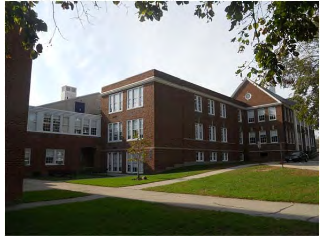
North and east elevations of B Wing
