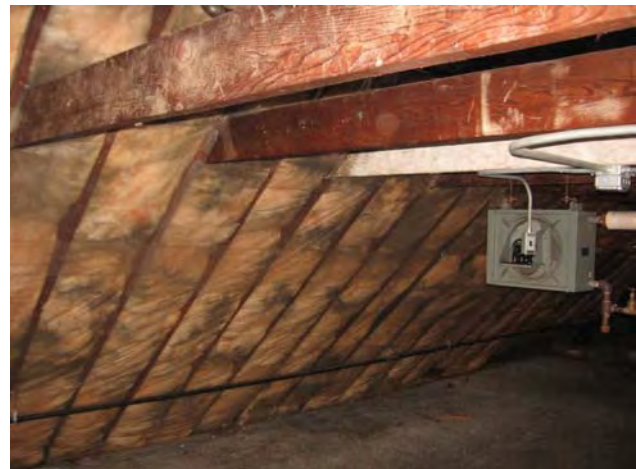
Conventionally framed gable roof over original flat roof (1931 renovation).
