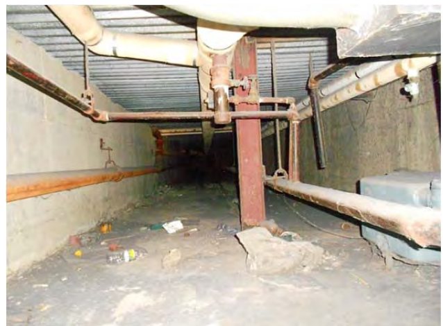
C wing crawlspace
