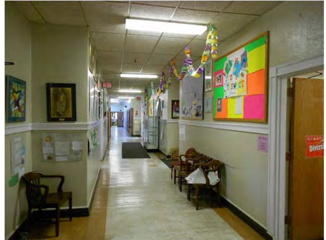
Interior walls of B wing are plaster
