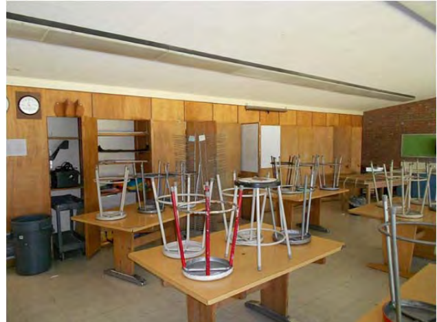
C wing casework is still serviceable but is nearing the end of its useful life
