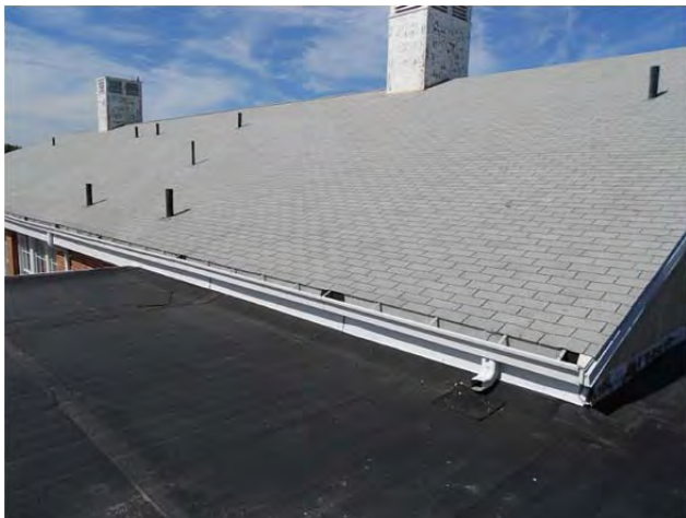
A wing transition to classroom wing shingled roof
