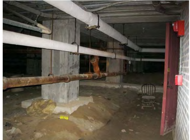
A wing crawlspace
