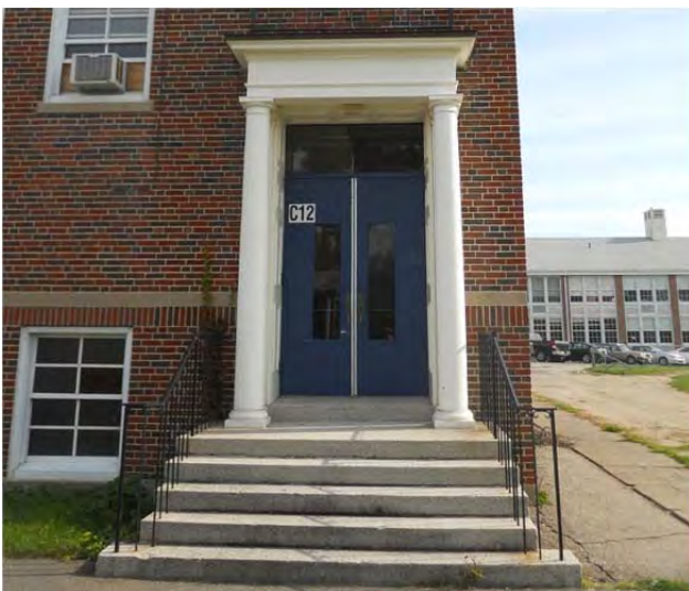
Portico elements of B wing's west side fabricated from GFRP
