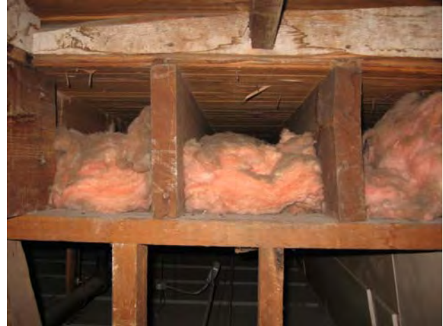
Wood joists supported on wood studs -typical floor framing at B-Wing (1917 Building).
