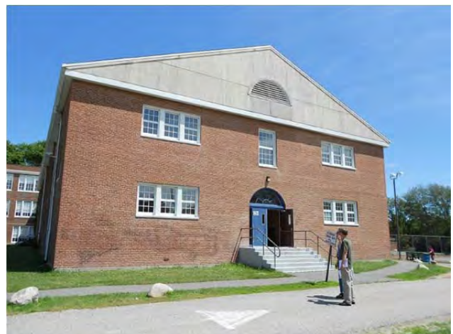
Stucco along the gable ends may conceal the original gable end
