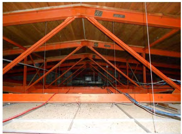
The above-ceiling space in C wing.
