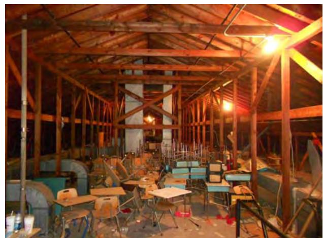
Conventionally framed gable roof above attic of classroom wing (A-Wing).
