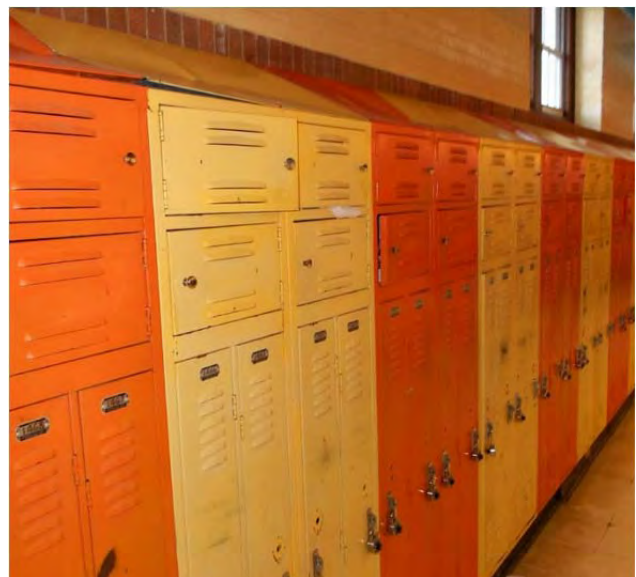
Sloped top lockers are used in B wing but retain the same narrow style as the rest of the facility.
