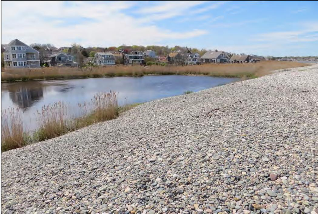
Figure 2.11 Overwash of beach material from Egypt Beach into Sheep's Pond creates large overwash fans (photo taken by Applied Coastal on May 10, 2016).
