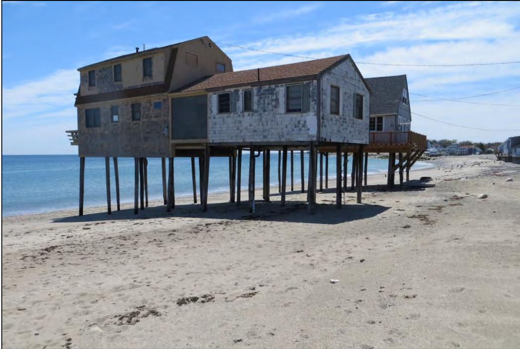
Figure 2.6 Dwellings along Town Way Extension, where the daily high tide line is under the buildings and the position of the houses is well seaward side of the low dune at Peggotty Beach (photo taken by Applied Coastal on May 10, 2016).
