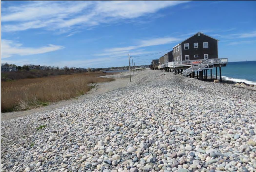
Figure 2.4 Dwellings along Stanton Lane illustrating proximity of the typical high tide line to the structures, as well as the position of the houses on the seaward side of the cobble dune crest (photo taken by Applied Coastal on May 10, 2016).
