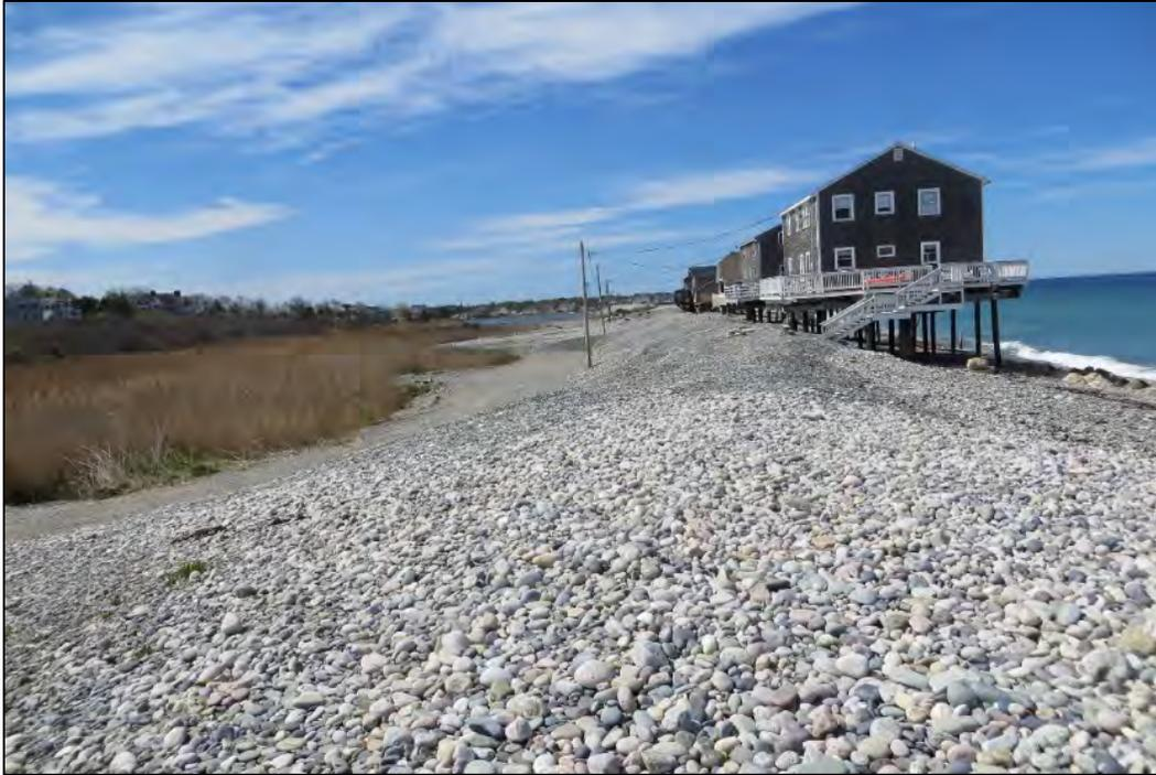
Figure 6.8 Mixed sediment dune at Mann Hill Beach, where the existing homes are located seaward of the dune crest (photo taken by Applied Coastal on May 10, 2016).
