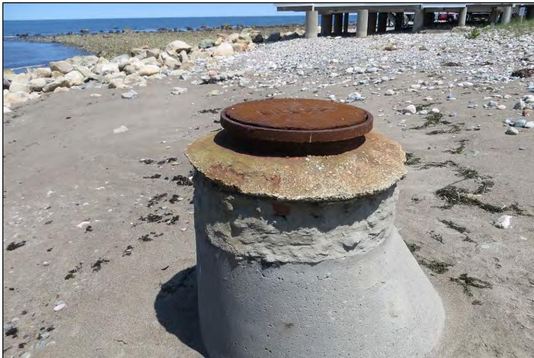
Figure 5.7 An exposed sewer manhole at Egypt Beach (photo taken by Applied Coastal on May 12, 2016).
