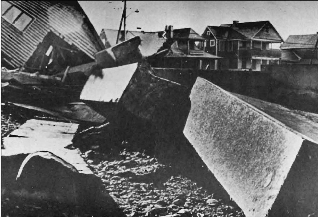
Figure 1.2 Portions of the North Scituate Beach seawall destroyed during the Blizzard of 1978 (image credit: *The Boston Globe*).
