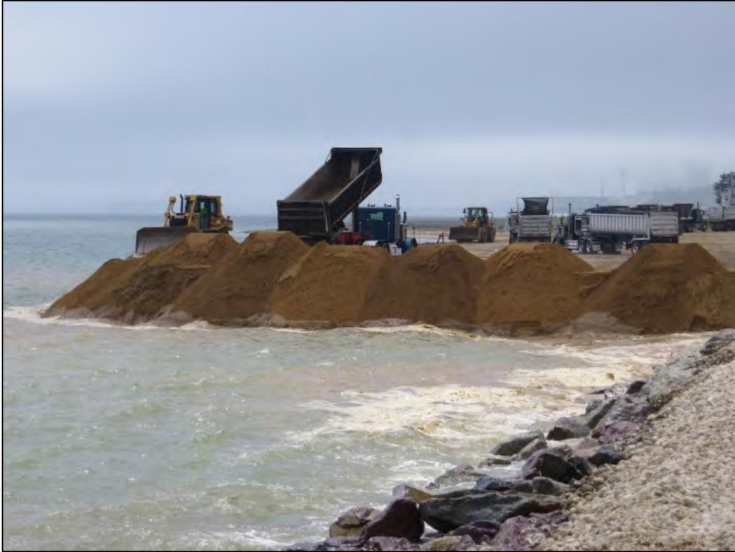
Figure 6.6 Placement of large-scale beach nourishment at Winthrop Beach, Massachusetts, where the designed beach berm was approximately 7 feet above the local high tide level (phot by Applied Coasta/).
