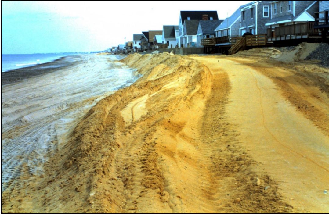
Figure 3.5 Placement of dune nourishment material along Humarock Beach in 1994 for the sacrificial dune project. ( Image source: CZM )
