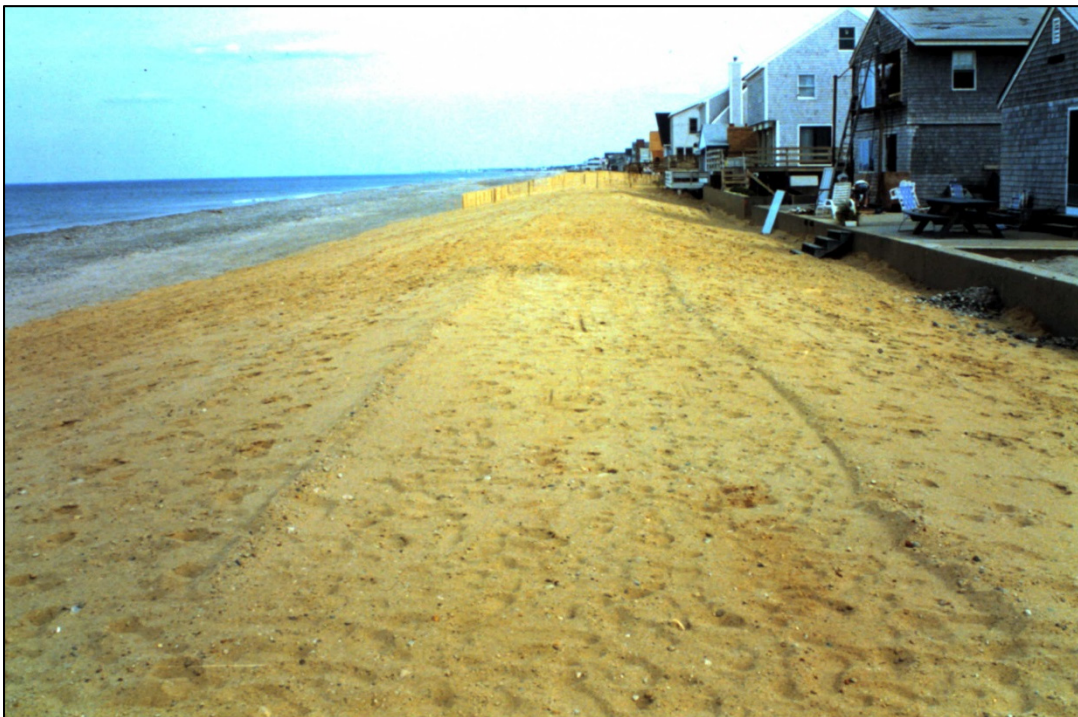
Figure 3.6 Constructed dunes along Humarock Beach in 1994 for the sacrificial dune project. ( Image source: CZM )
