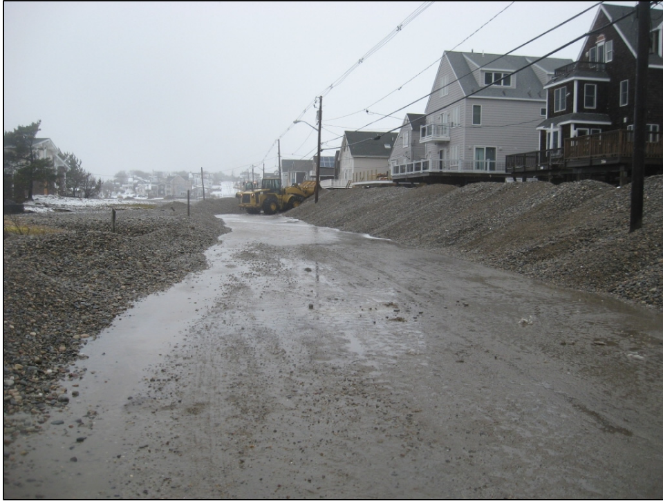
Figure 2.3 Road clearing efforts along Central Avenue. Overwashed sediment is piled along the sides of the road. (Image source: Jason Burtner on March 8, 2013)
