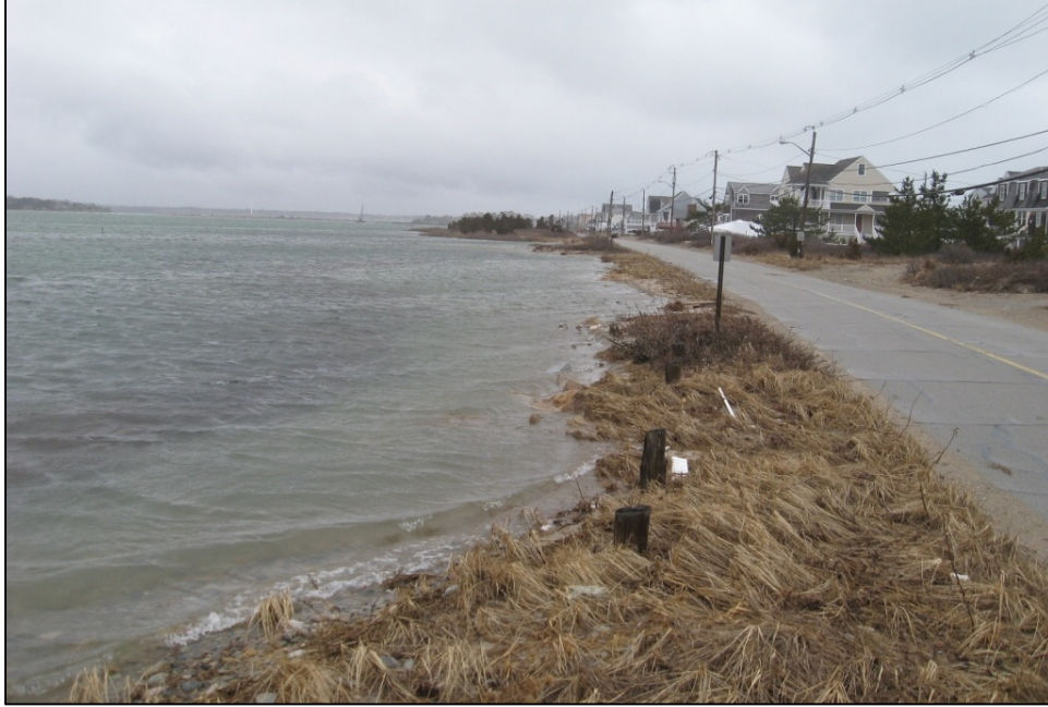
Figure 2.6 Near-flooding conditions at Central Avenue on where the water level is approximately 6.5 feet NAVD88. ( Image source: Jason Burtner on March 31, 2014 )
