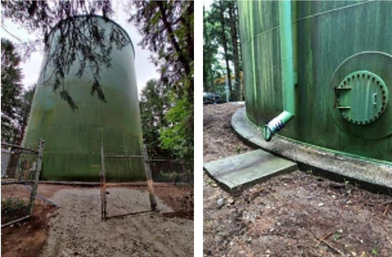
This site consists of the Mann Lot Road standpipe located in a wooded parcel. The tank is enclosed by a chain link fence with a double-leaf gate and barbed wire. A pressure transducer was recently installed.
