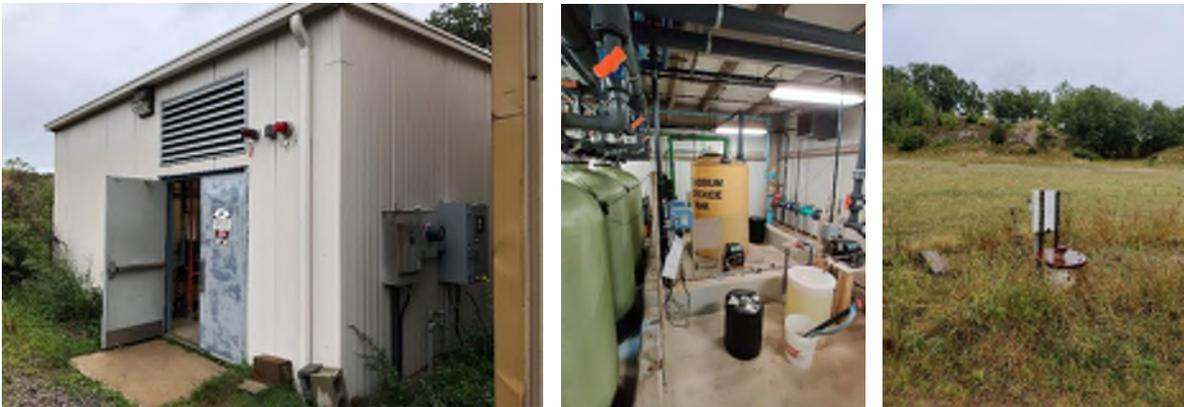
This facility was built in approximately the 1990's. The onsite yard is shared with the transportation department. Sodium hypochlorite is added to disinfect the raw water and potassium hydroxide is added to adjust pH for corrosion control. A fluoride system is in place but is currently inoperable and in need of repair or replacement.
