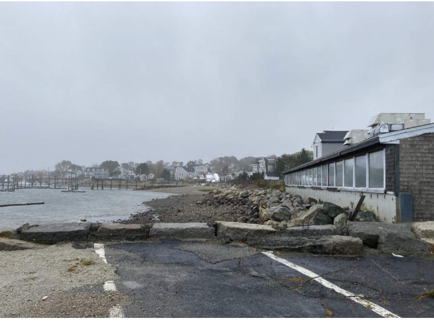
GRANITE SEAWALL / BUILDING FACE TRANSITIONING TO RIPRAP / VEGETATION (LOOKING SOUTH)
