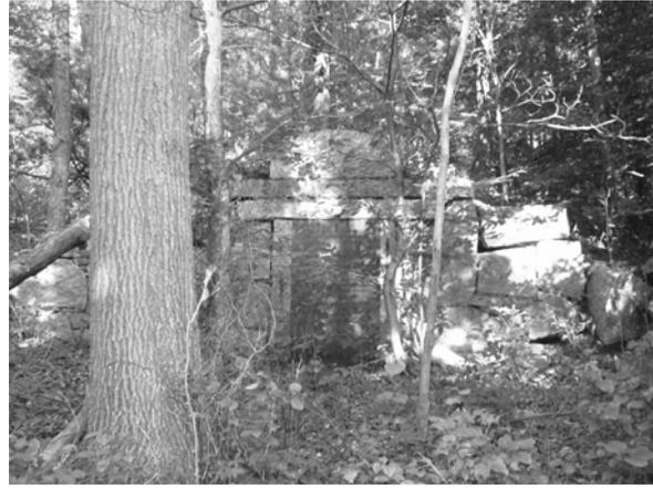
The tomb structure rests against a hillside, is constructed of cut granite, and is in fair to poor condition. The front wall has moved and the right cheek wall has failed, with stones missing. Deciduous trees have volunteered in and around the tomb, contributing the structure's deterioration. One tree has fallen on the tomb to the left of the door. While the door has been sealed with mortared brick, hardware remaining in the door jam area suggests the tomb once had a door.
