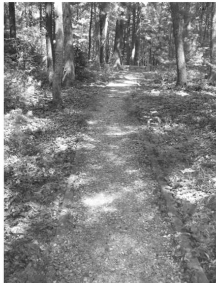
*The existing pathway to the Cushing Family Cemetery is lined with wood timbers. These should be replaced with granite edgestones as they rot.*
