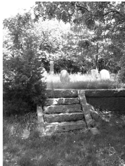
The overall condition of the wall and steps is very poor. The wall is significantly bowing, with a bow greater than two inches in most locations. Many small trees and shrubs have volunteered in and around the wall, further compromising the strength of the wall. It is likely that the original wall was dry laid, and that mortared was added at a later date, trapping water behind the wall
