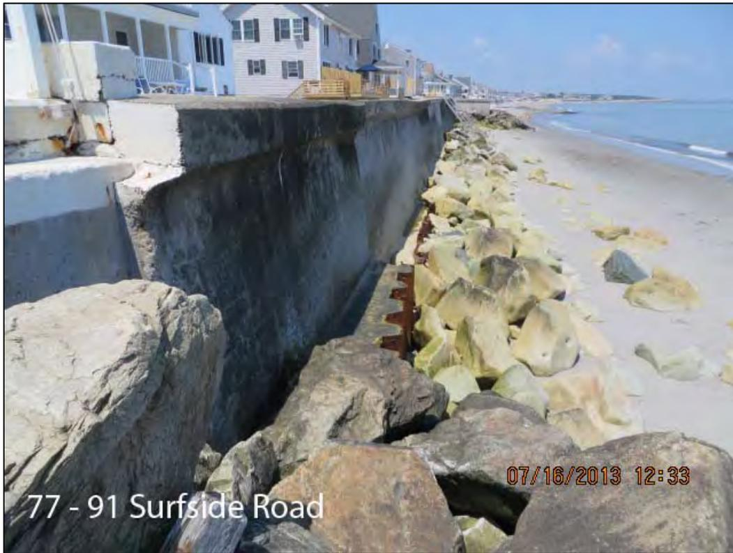
Figure 7.11 Existing seawall and revetment along Surfside Road (photo by CLE Engineering).
