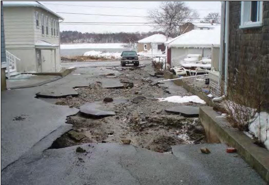
Figure 6.4 Damage to pavement caused by wave overtopping in Hull, MA (photo credit: MCZM).
