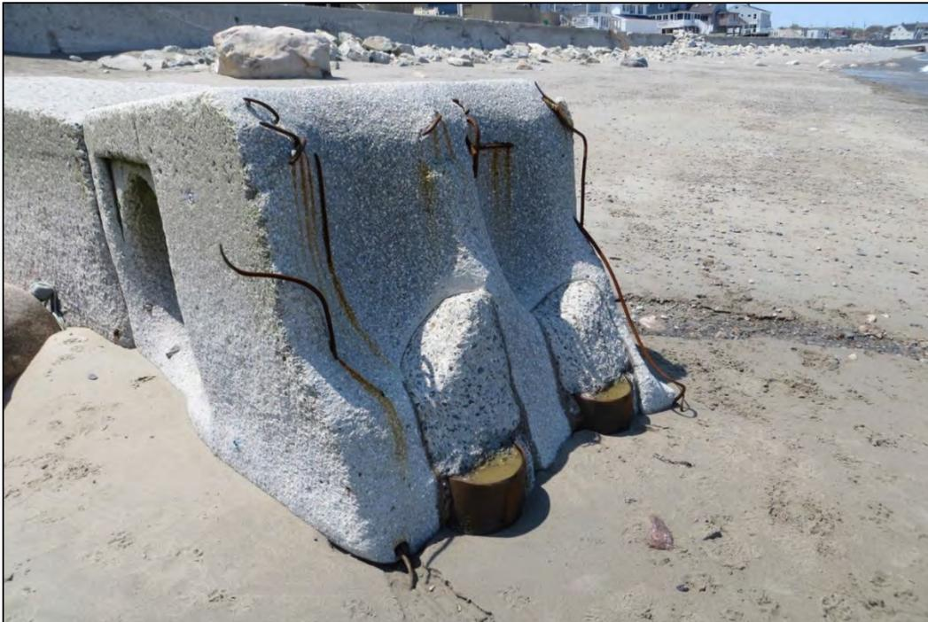
Figure 6.21 Observed scouring of concrete surface of outfall structure along Oceanside Drive. It is anticipated that degradation of concrete would be more rapid along the cobble/boulder strewn platforms at Cedar Point or Egypt Beach.
