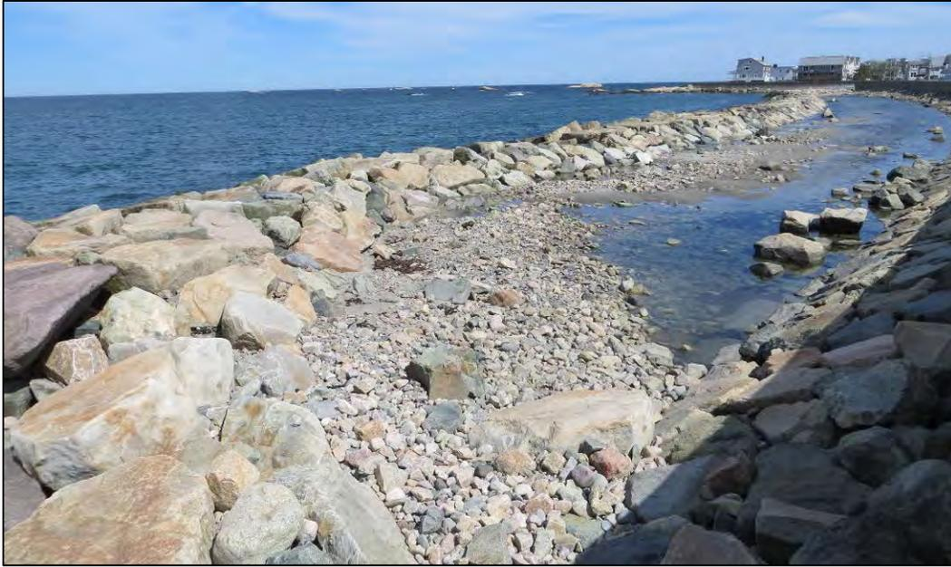
Figure 7.3 Existing revetment dike at Minot Beach (photo taken by Applied Coastal on May 10, 2016).
